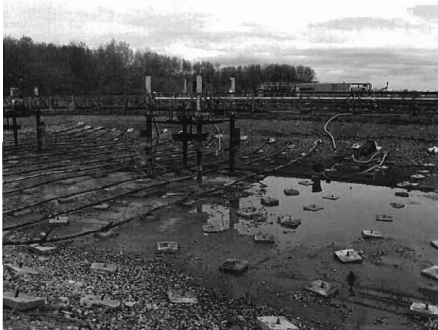
May 4, 2010 Dewatering and Piping/Concrete Anchor Removal
