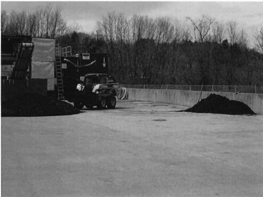
April 9, 2010 Sludge Stockpile Containment Area – Concrete Drying Bed
