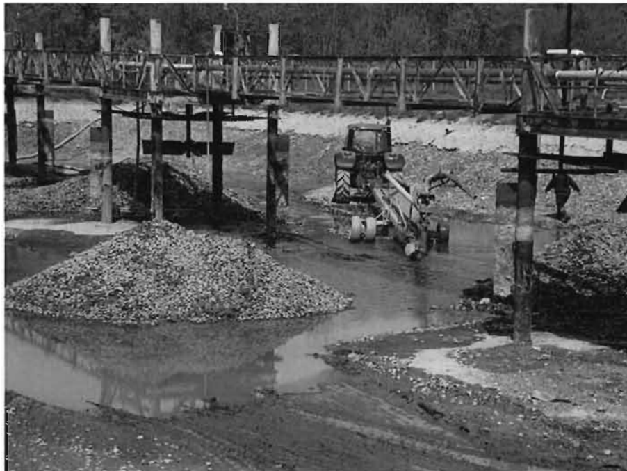
May 11, 2010 Aeration Basin Sludge Removal
