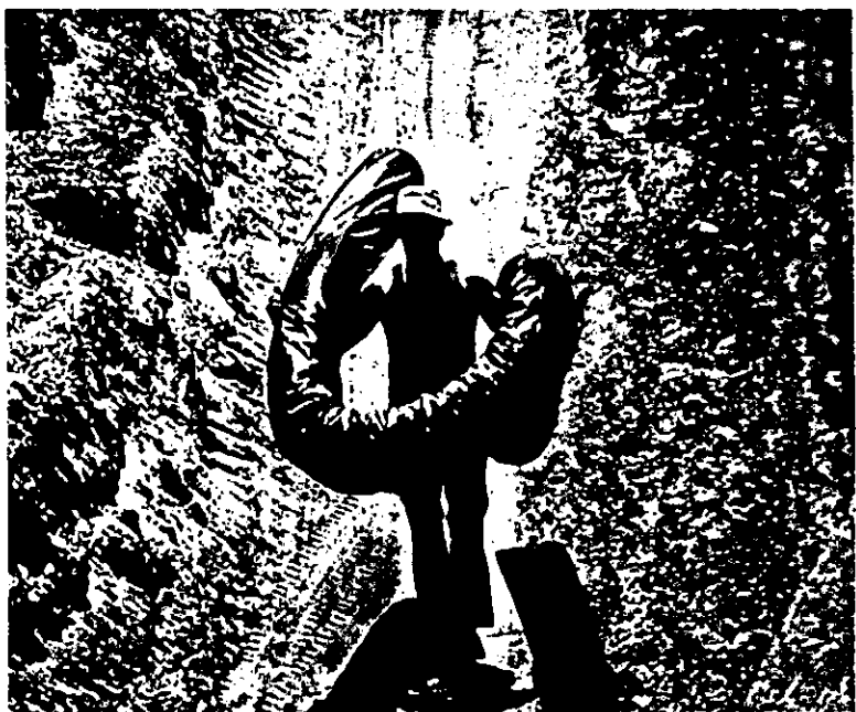
■ BEDDED on stone, pipe was covered with pervious gravel to surface. Plastic wrapping provided ultraviolet protection during outside storage.
