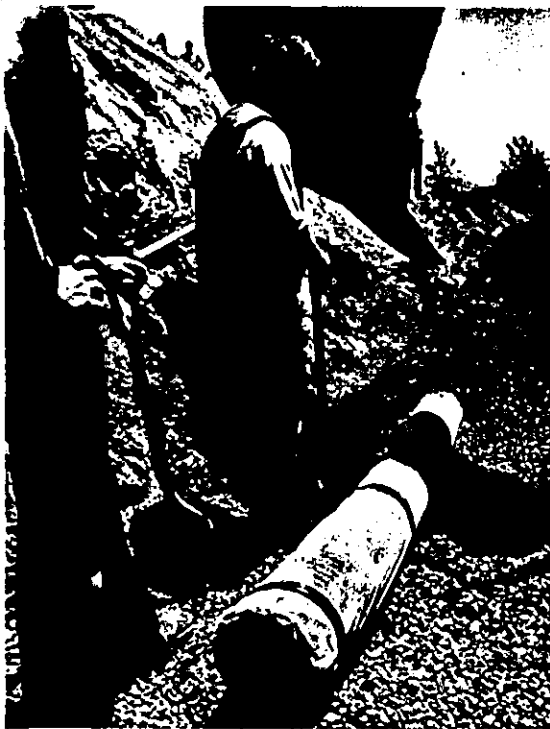
■ BEDDED on stone, pipe was covered with pervious gravel to surface. Plastic wrapping provided ultraviolet protection during outside storage.
