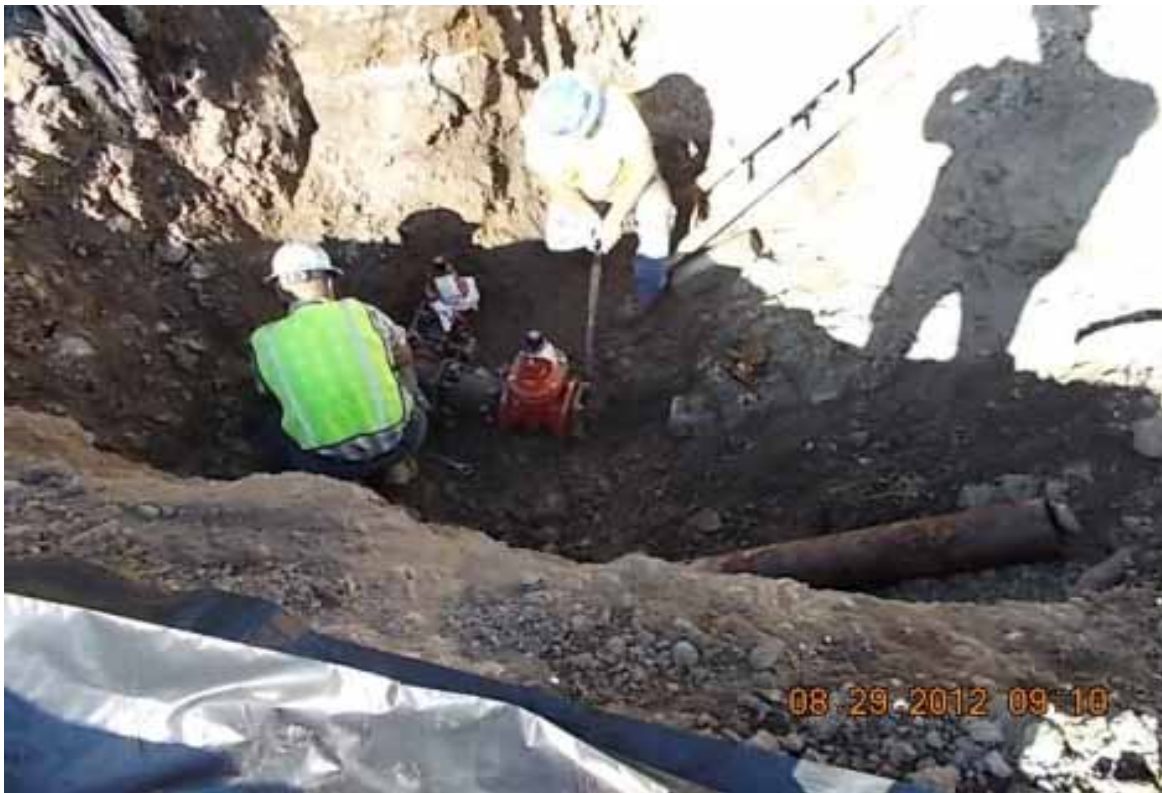
Photo #1: Installing water main shutoff valve and tee for the grout batch plant water supply line (Approximately 10 feet southeast of monitoring well MW-11)
