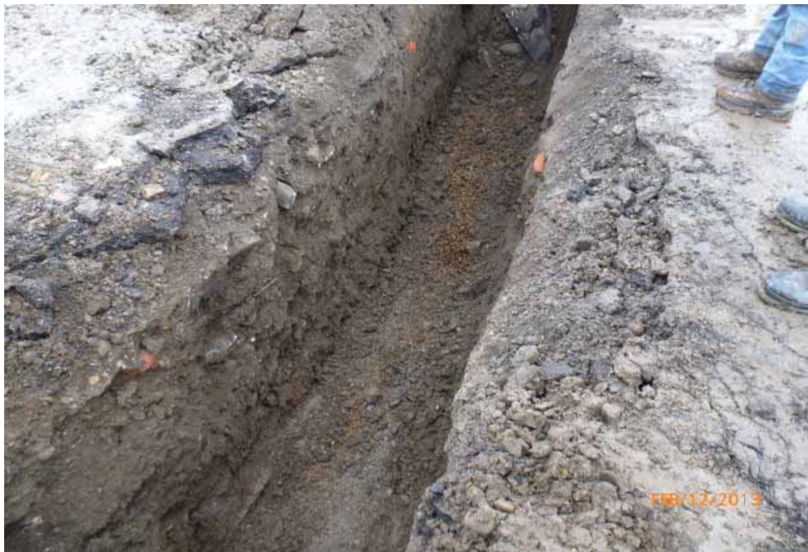
Photo #8: Backfilling of water main installation trench
