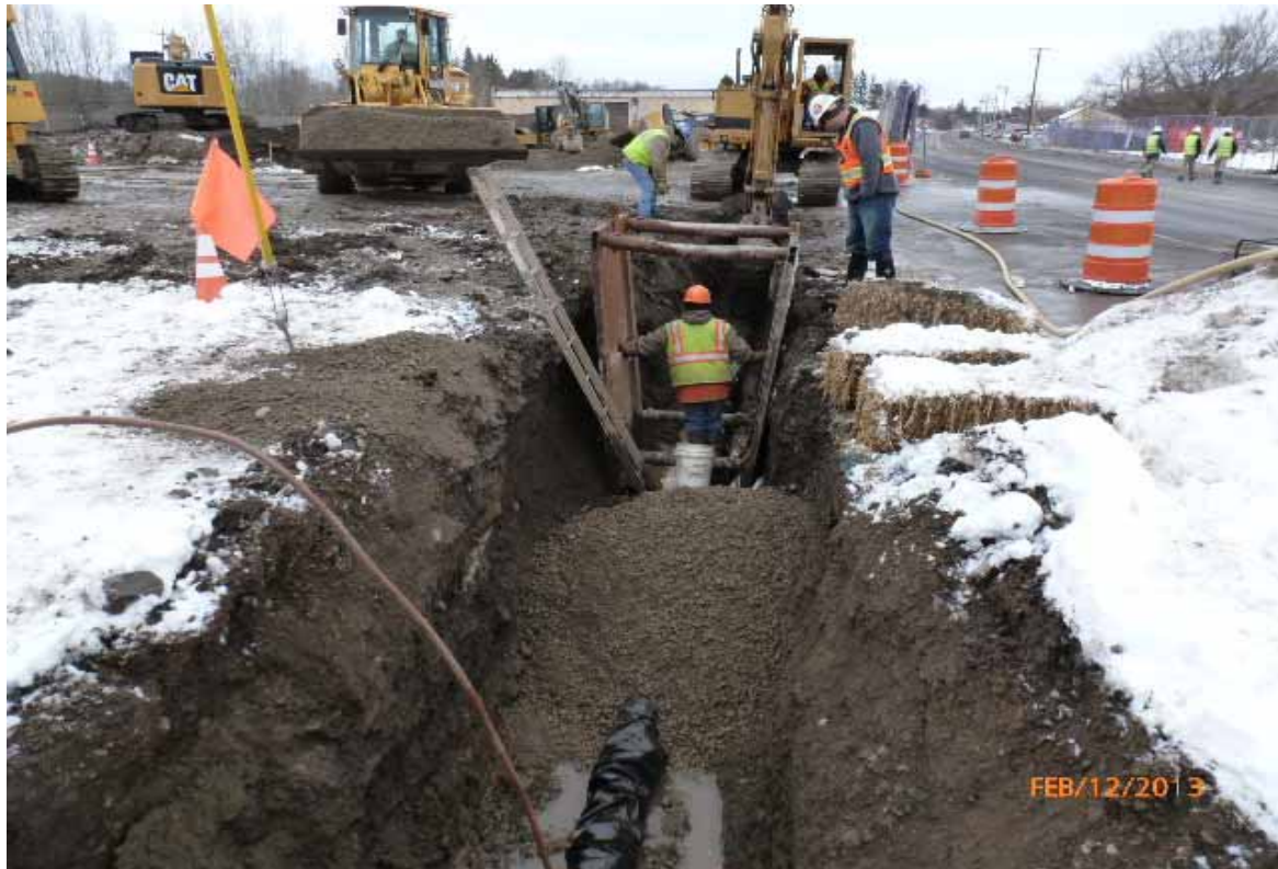
Photo #7: Water main installation trench (additional view)
