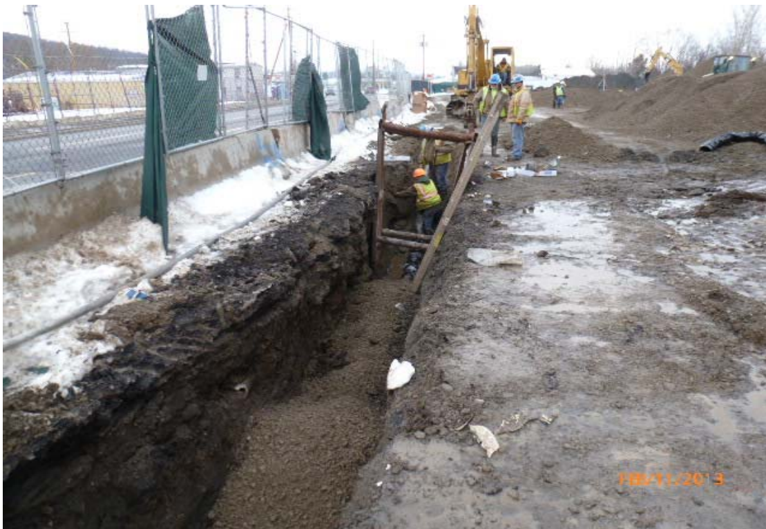
Photo #16: Water main installation trench continuing south.
