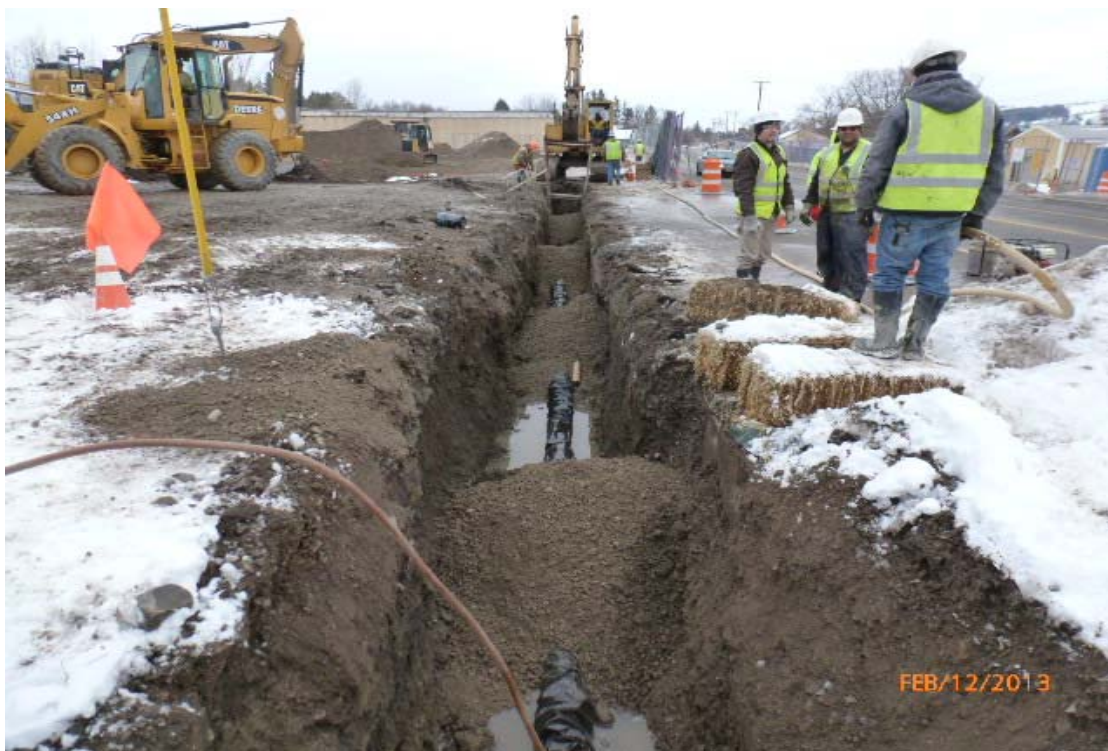
Photo #23: View of pipe with wrapping and stone bedding.
