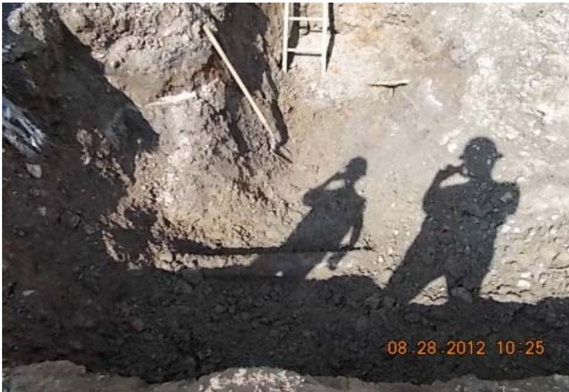
Photo #8 Water main excavation for installing new fire hydrant.
