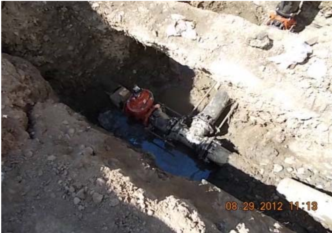
Photo #7: Installing water main "T".
