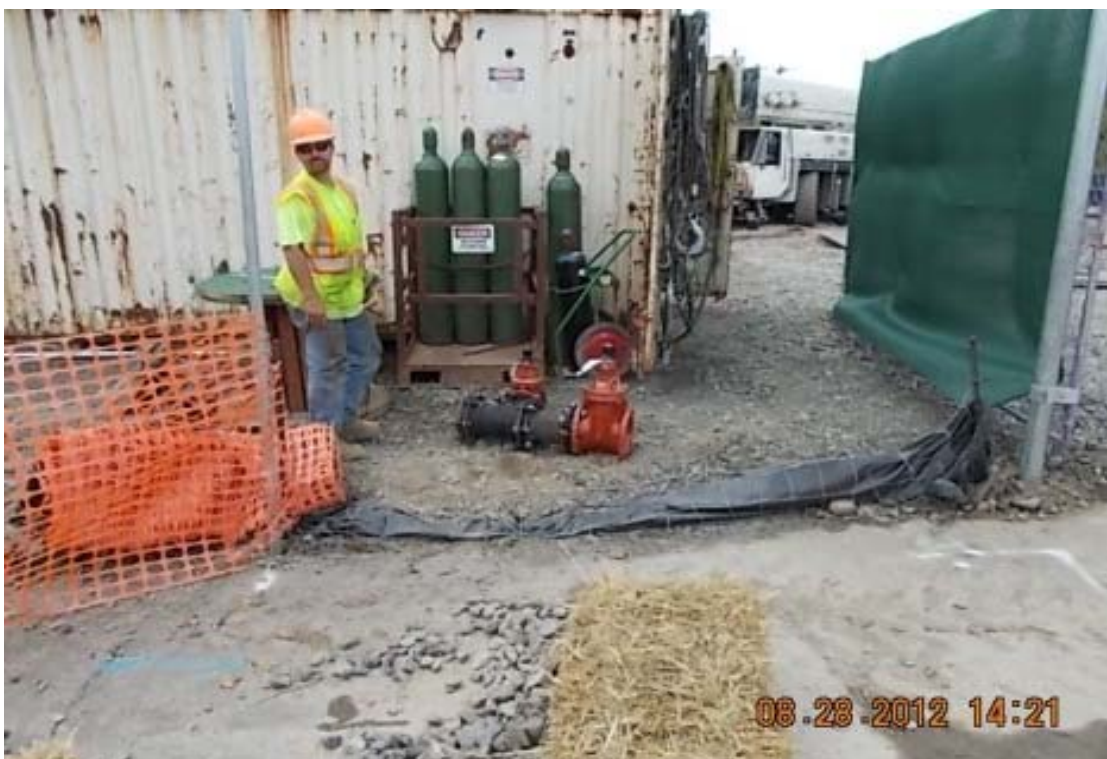
Photo #6: New water maint "T" for water supply.
