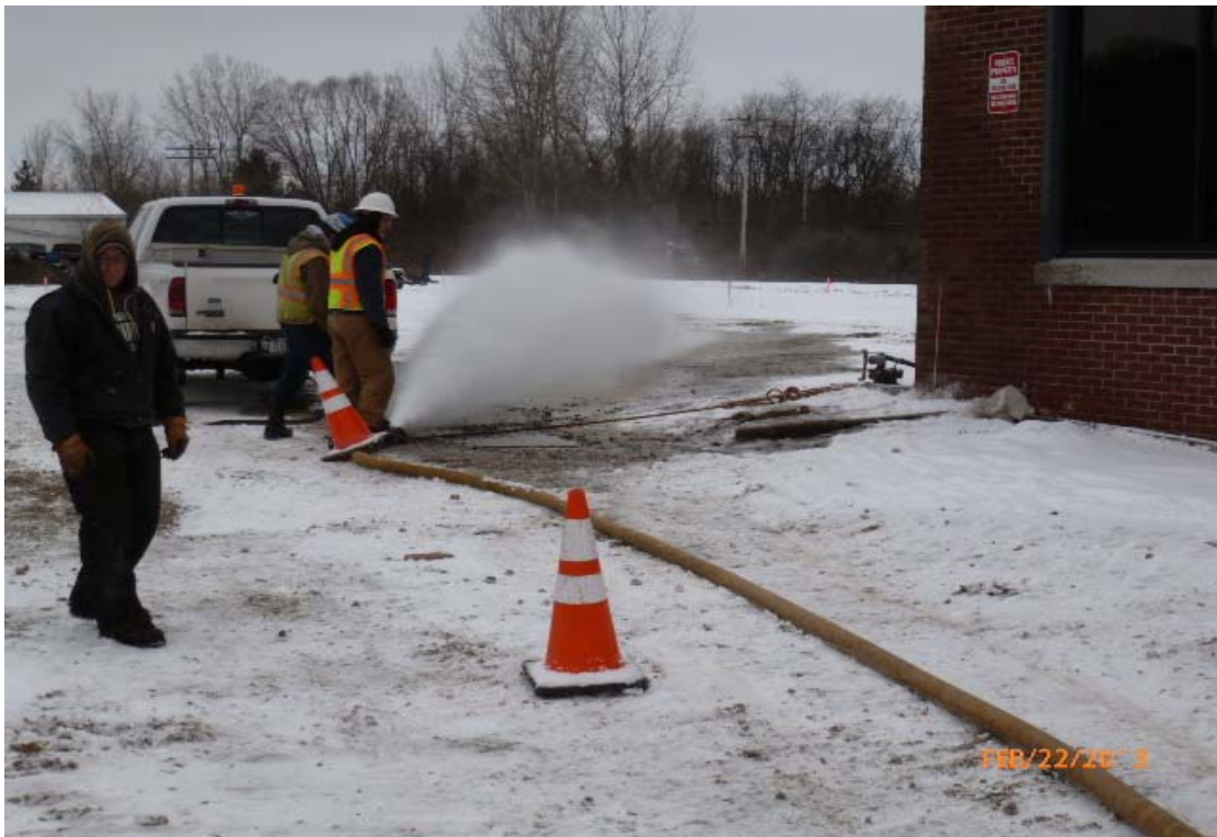
Photo #28: Grant Street and the Village of Homer flushing the water line.
