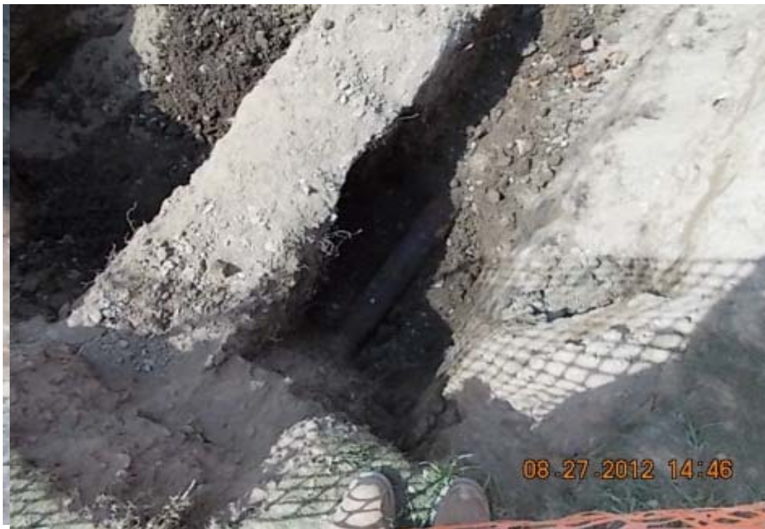
Photo #4: Exposed original water main.
