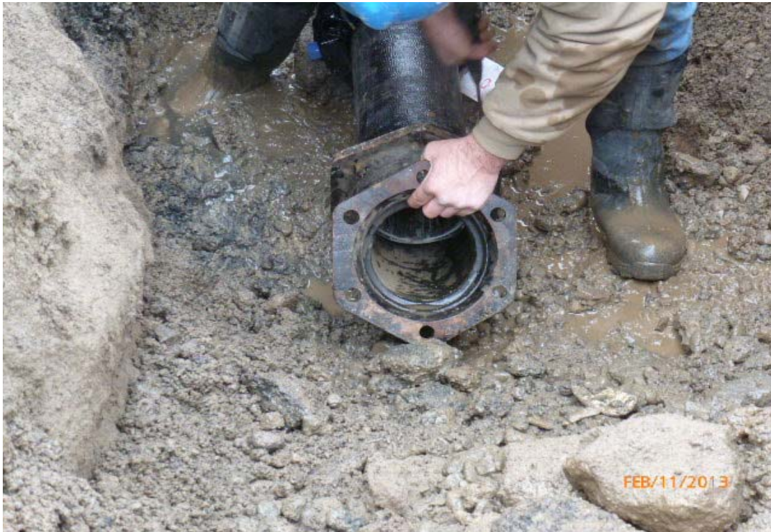
Photo #15: View of 45-degree fitting to bring water line above monolith.
