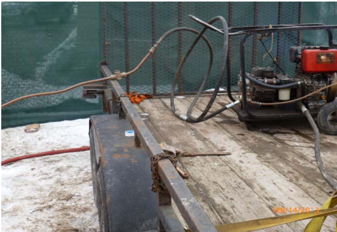
Photo #26: Pump used to add chlorinated water to the new water main.
