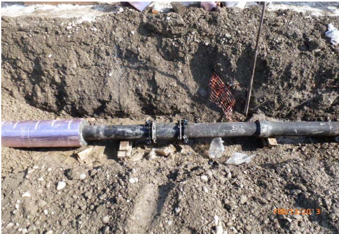
Photo #20: View of coupling in center of monolith.
