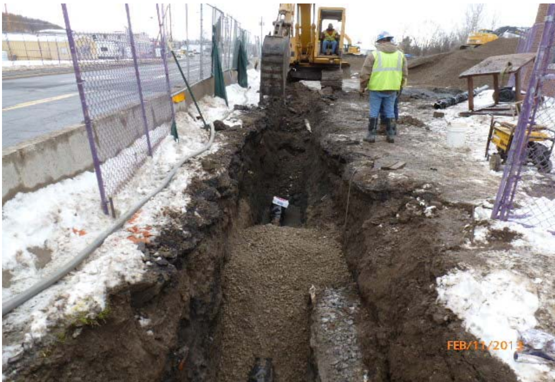
Photo #22: View installation trench continuing south.
