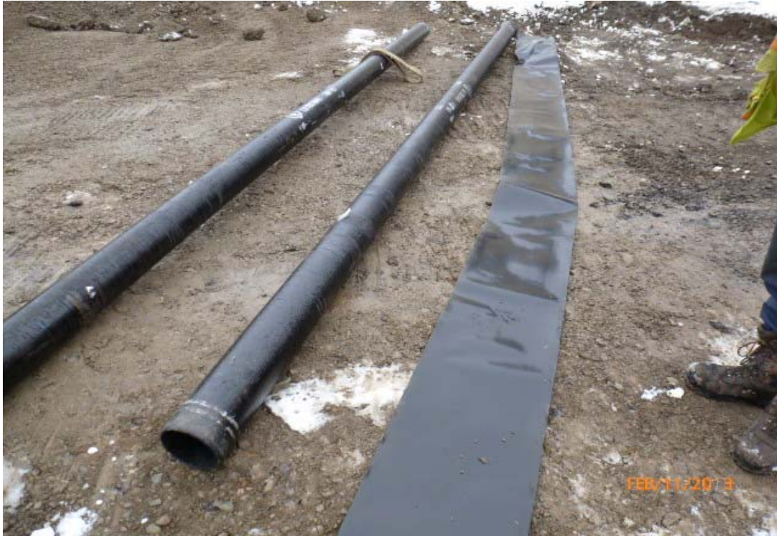
Photo #11: View of new water main to be installed and pipe wrapping.
