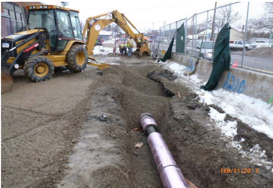
Photo #18: Backfilling and compacting portion of water main installed over the monolith.
