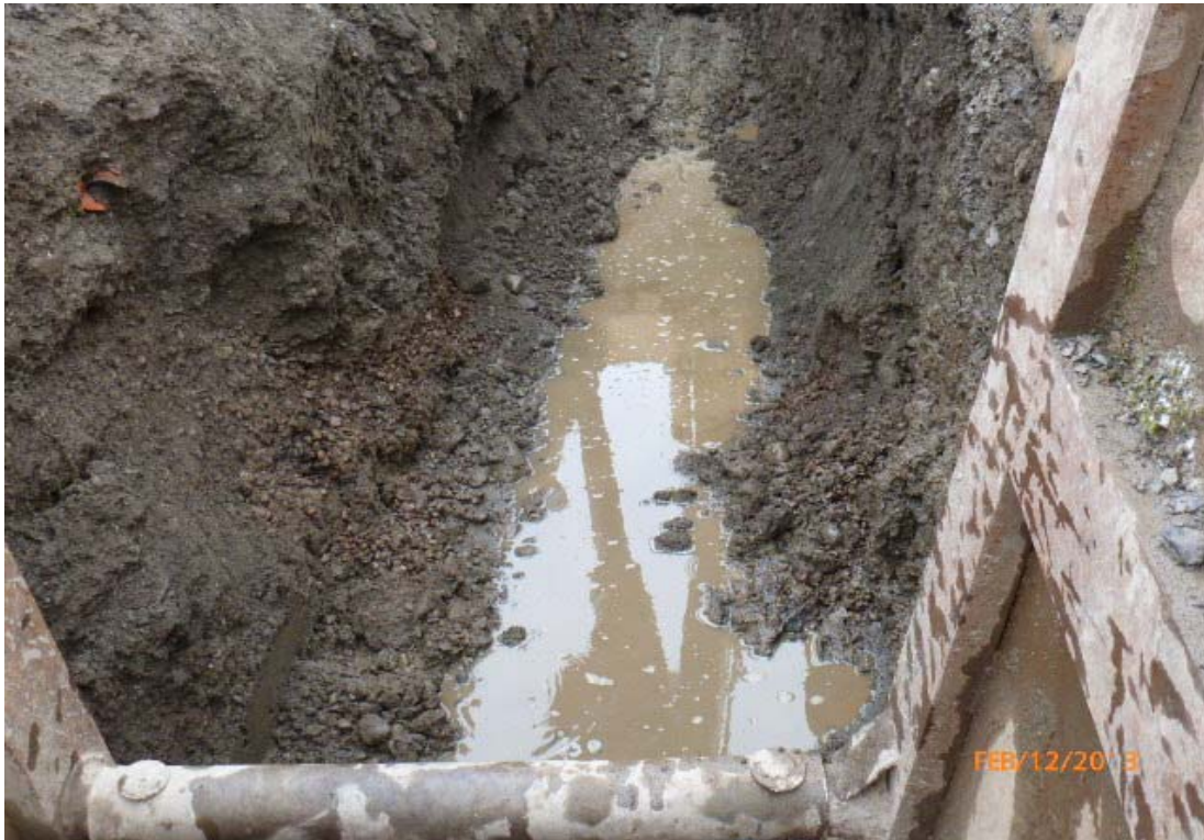
Photo #25: View of water in trench one hour after being excavated.
