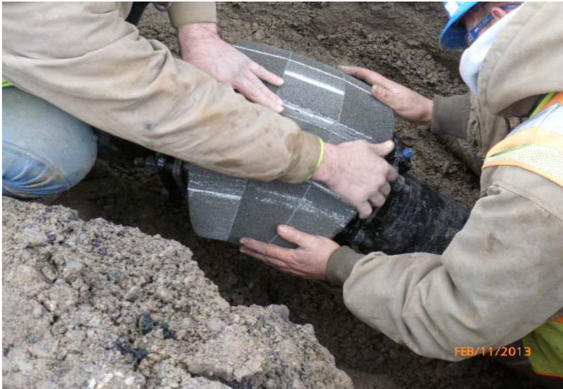
Photo #21: Installation of insulation on 45 fitting.
