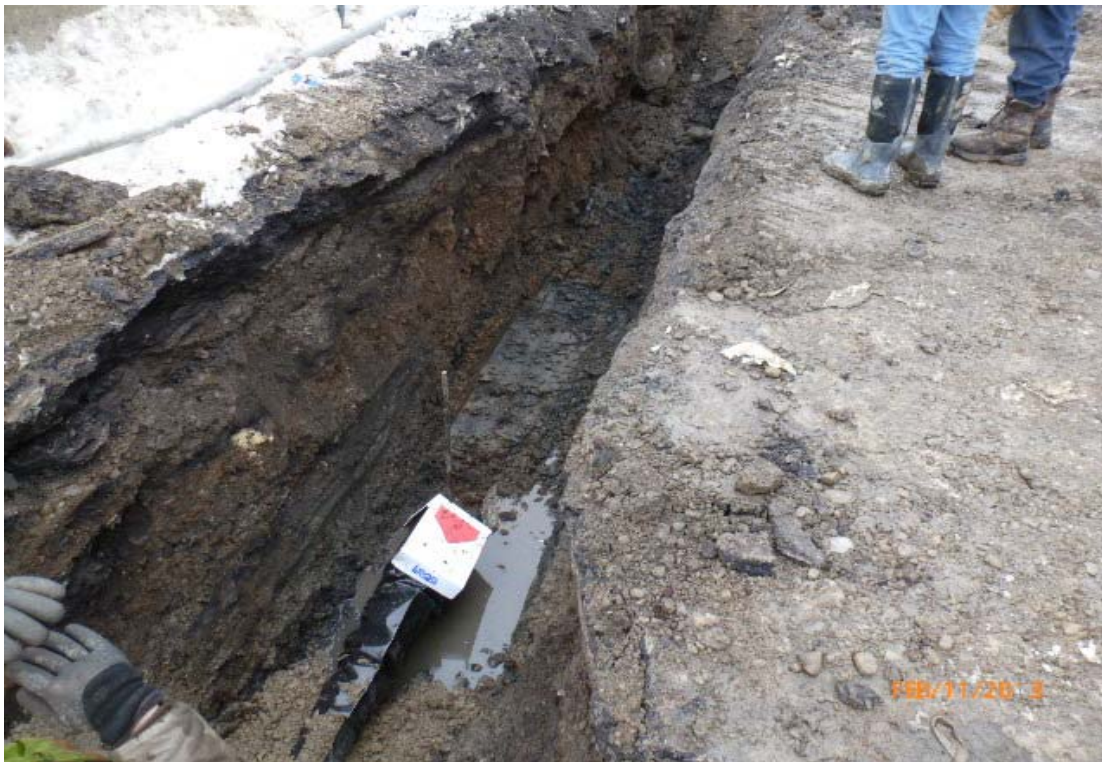
Photo #12: View installation trench continuing south.
