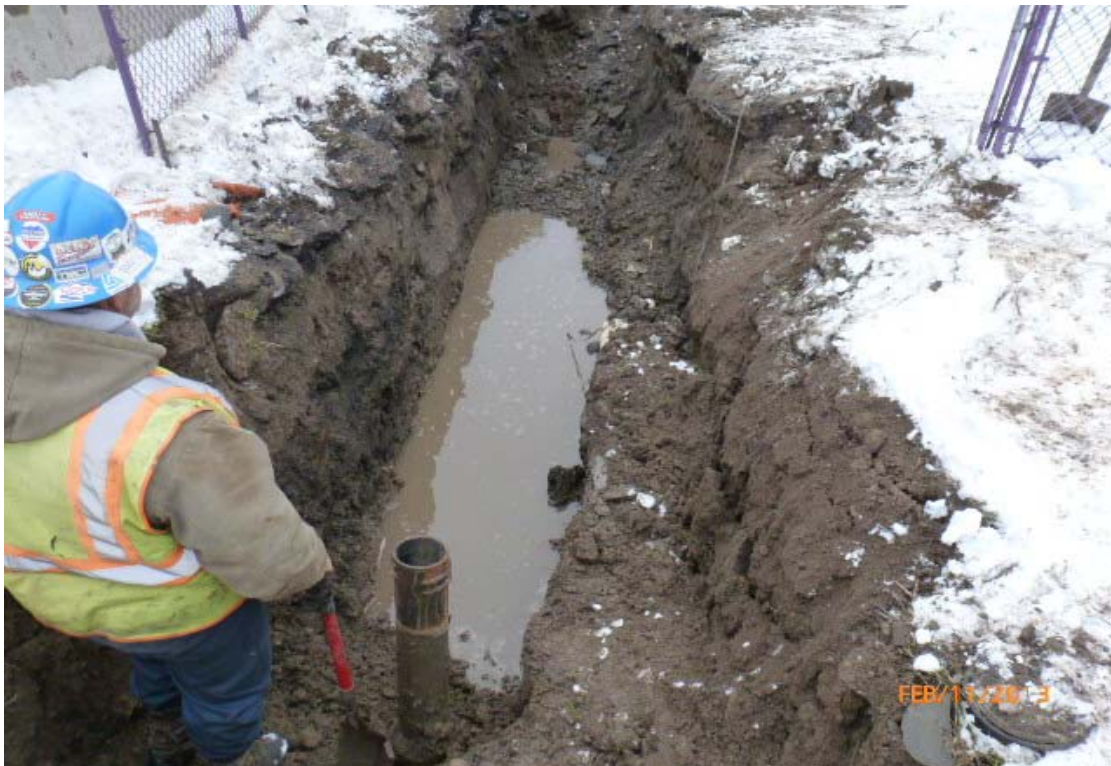
Photo #10: Start of excavation for new water main installation at ID Booth.
