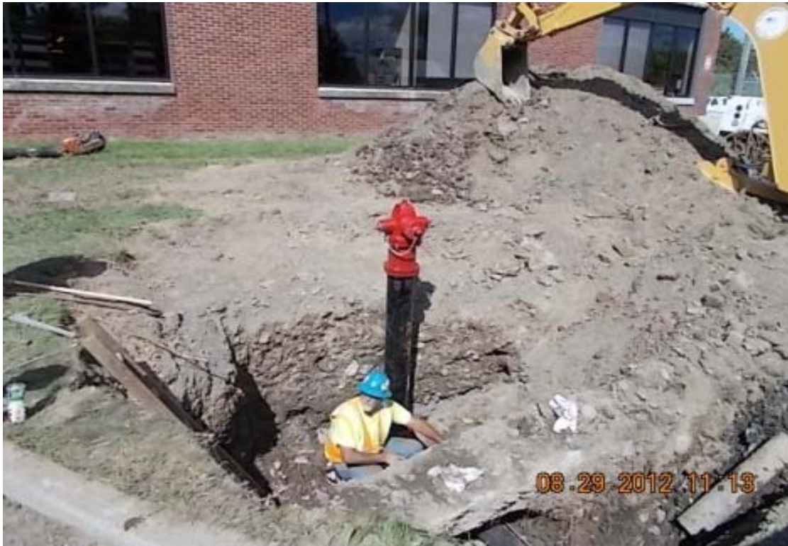
Photo #9: Installation of the new fire hydrant.
