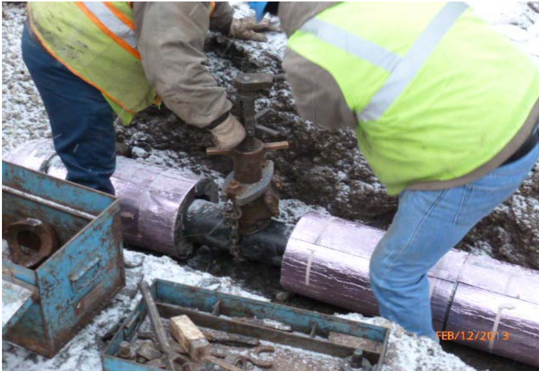
Photo #19: Installation of tap to 2" line for chlorination/testing (north end).
