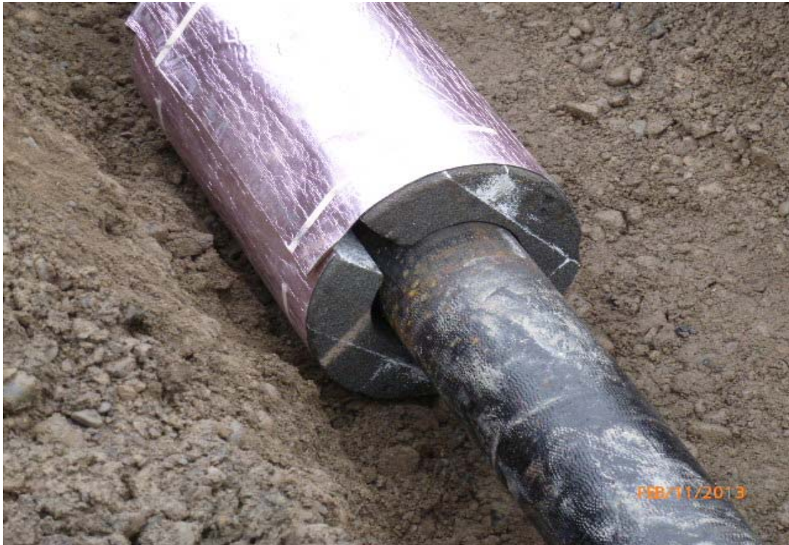
Photo #17: Insulations used where the pipe is above the monolith.
