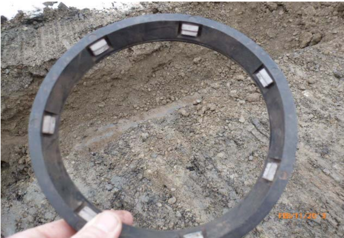
Photo #14: Field lock restraint used adjacent to 45-degree vertical bends.
