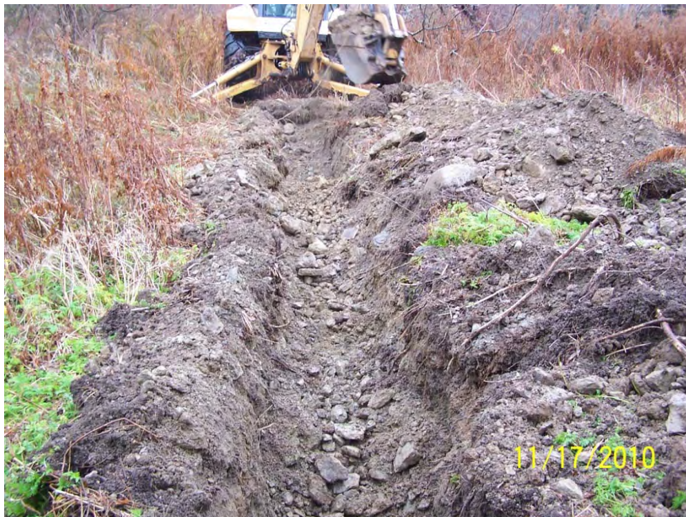
Photo 7585. TP-3, looking toward landfill from toe of slope (South Hill Road). Test pit uncovered shallow weathered bedrock. Waste located approximately 80 ft from toe of slope.
