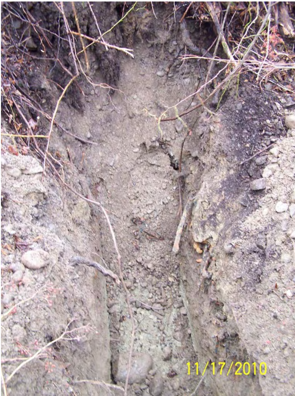
Photo 7603. TP-4 looking toward slope, which contained sand and gravel. At the toe of the slope there was a thin layer of solid waste, visible on the right side of this test pit.
