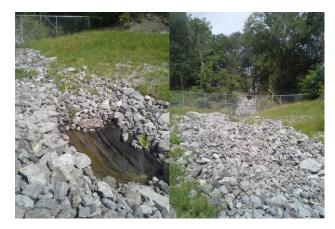
Aztech performed repair activities to several sections of the drainage swale at the site. Misplaced rip-rap from excessive storm water runoff at the site, was relocated back on top of exposed geotextile, as shown in the before and after pictures to the left. Rip rap was relocated by hand from areas downstream of the exposed areas, placing larger stones first then smaller stones. Several exposed areas were discovered and repaired in addition to the two areas described in the SOW.
