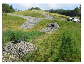
The detention pond outlet structure is shown in the photograph to the left and a detailed drawing is attached to this document in **Figure 3**. The cap to the outlet structure was removed and a 15" diameter hole was cut into the top of the cap to allow for overflow to be able to
