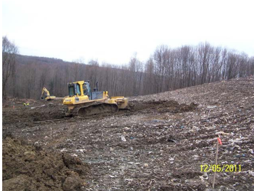
Landfill Subgrade Preparation, looking South
