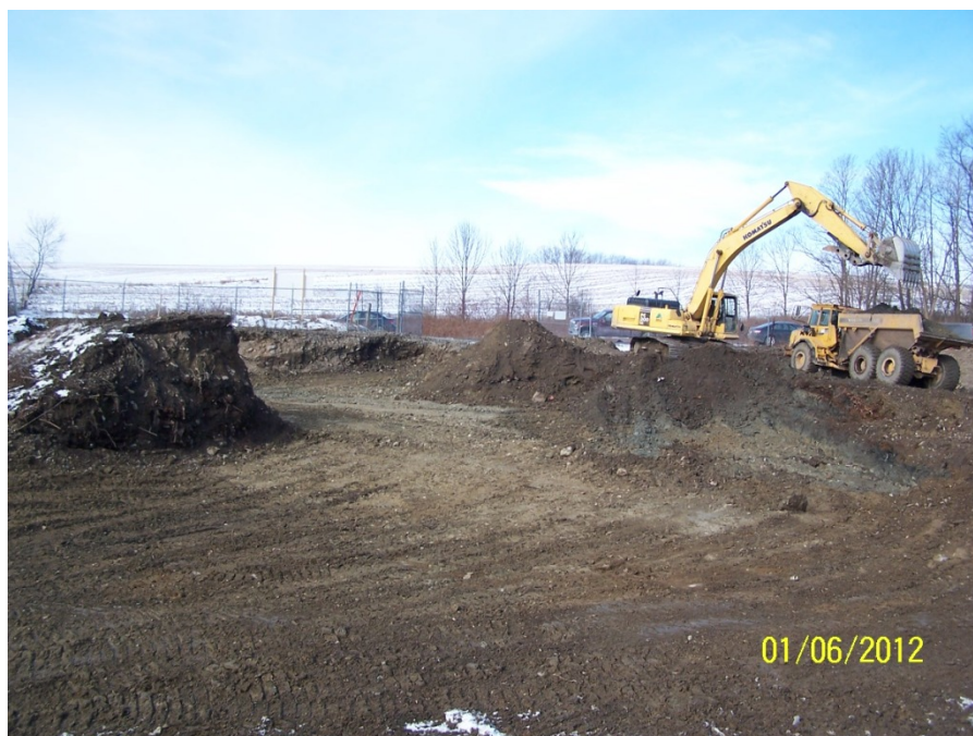
Excavation at the Former Parking Area, Looking Northwest
