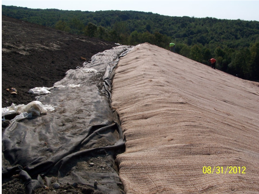
Laborers Installing Erosion Control Blankets on the Landfill Slope, Looking Southeast
