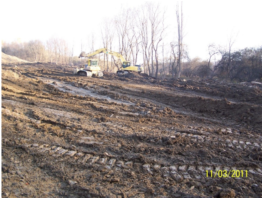
Consolidation of Waste Soil, Looking East
