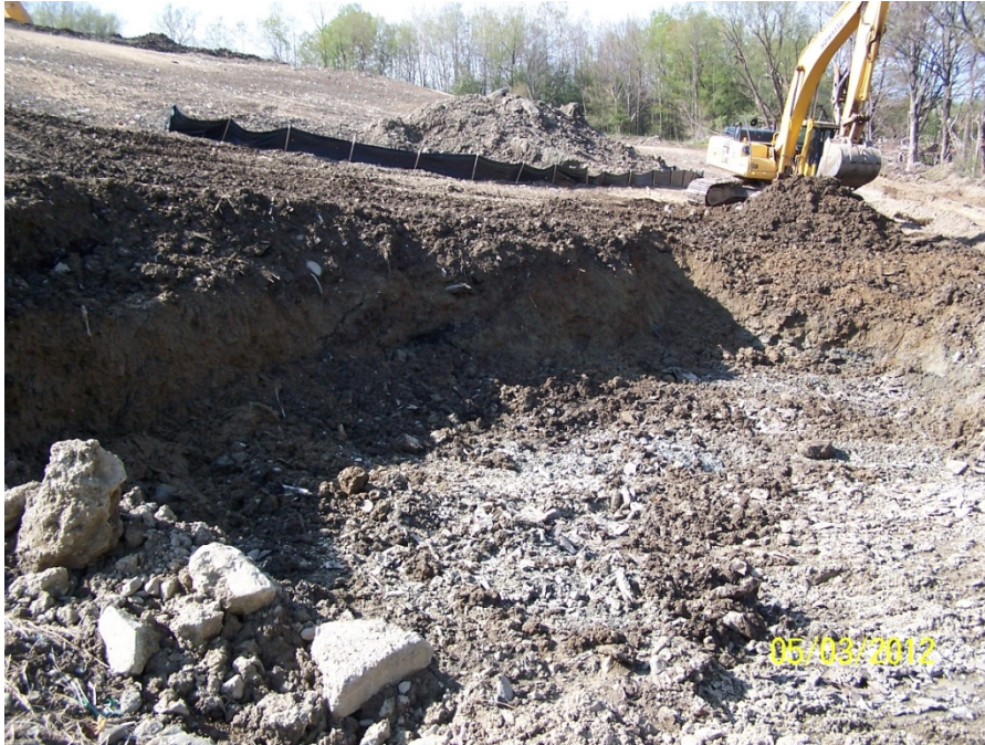
Excavation of Soil at Groundwater Seep, Looking North
