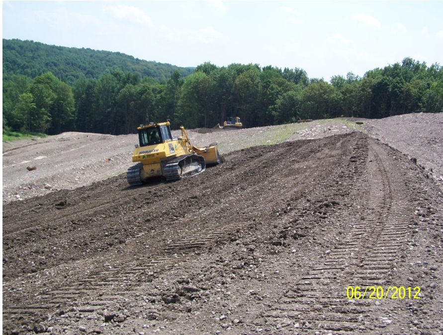
Placing and Grading Cover Soil on the Landfill, Looking Southeast
