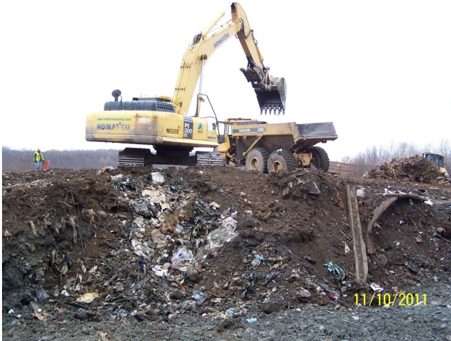
Solid Waste Consolidation (3), Looking South
