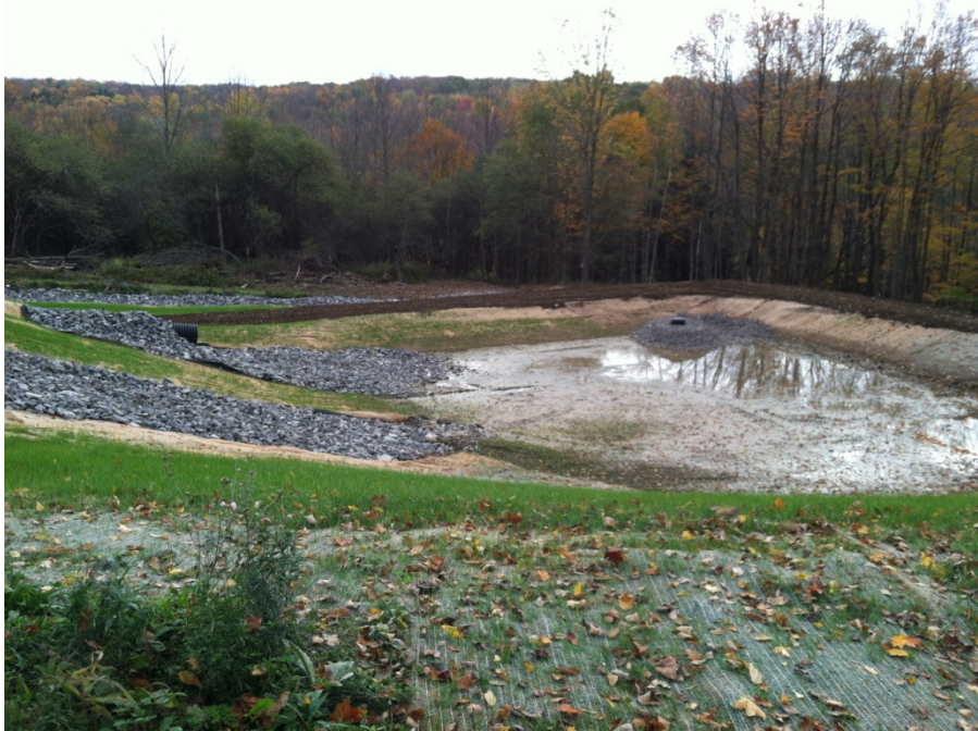
Detention Basin, Looking Southeast
