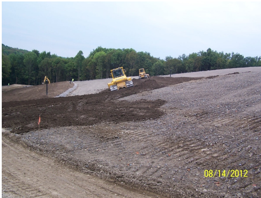
Placing and Grading Topsoil on the Landfill, Looking Southwest
