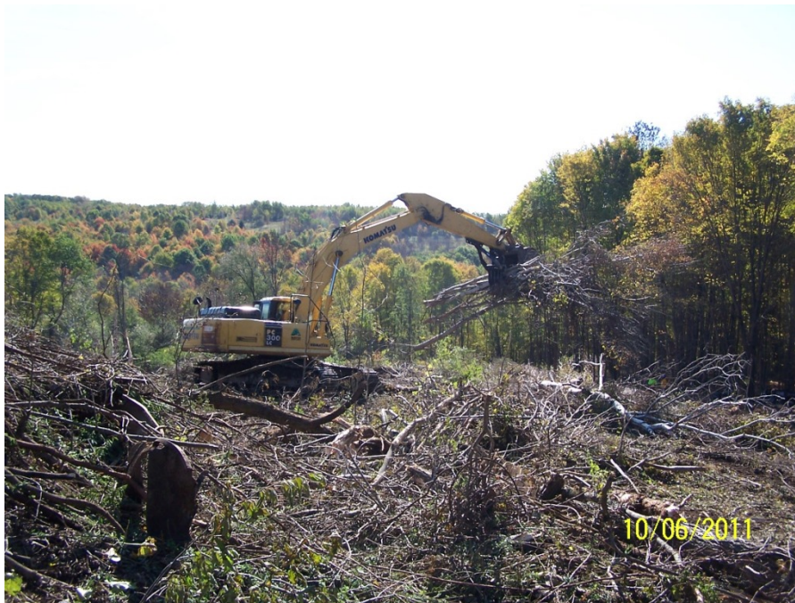
Excavator with “Thumb” Attachment, Stacking Cut Trees and Brush, Looking Southeast
