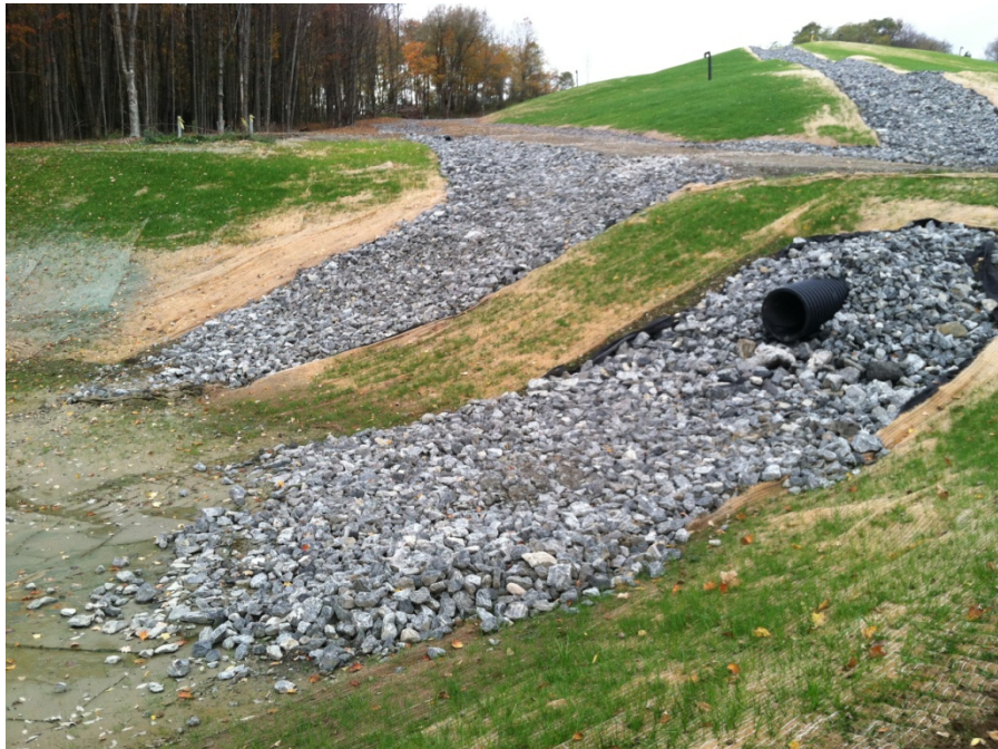
Culvert and Rock Outlet Protection at the Detention Basin, Looking Northwest
