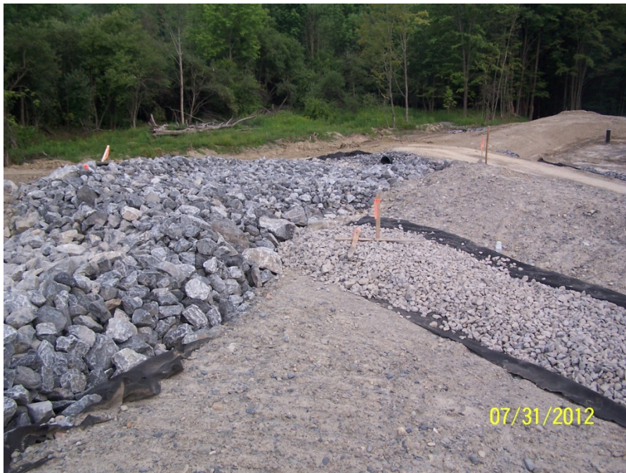
Rip Rap Installed at the Downdrain and the Bottom Slope Bench on the Western Side, Looking Southeast
