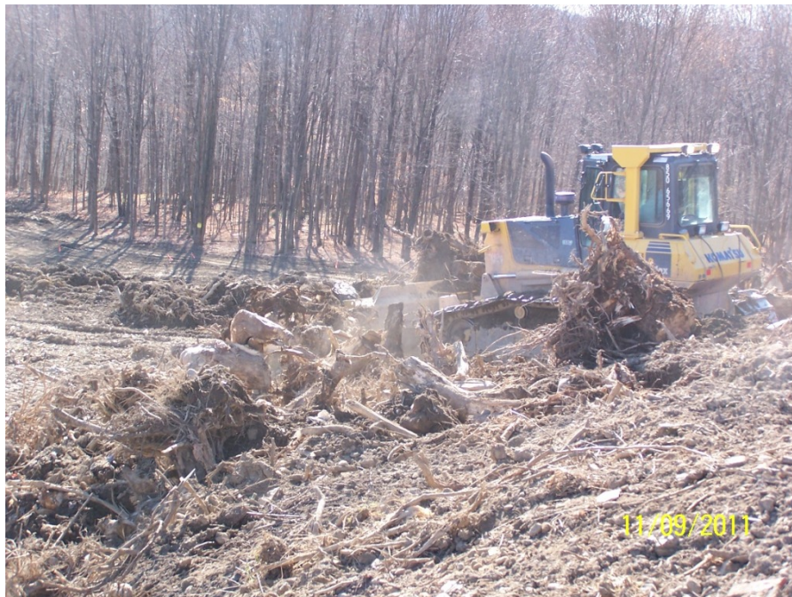
Dozer Tracking Grubbings during Placement within the Landfill Limits, Looking South
