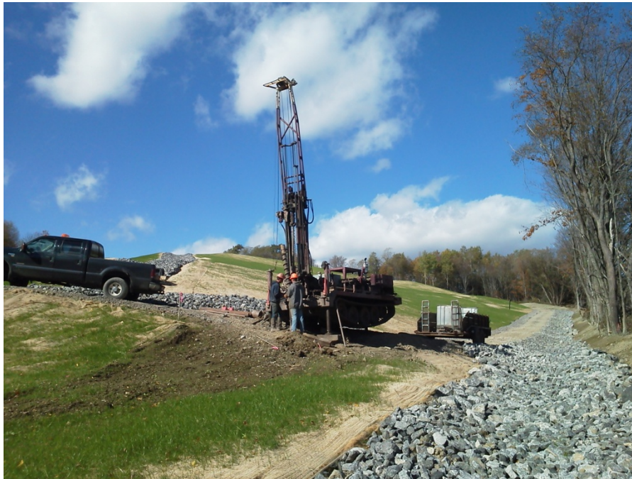
Installing Replacement Groundwater Monitoring Wells, Looking Northwest
