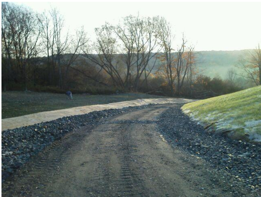
Eastern Perimeter Access Road, Looking Southeast Along Eastern Edge of Landfill
