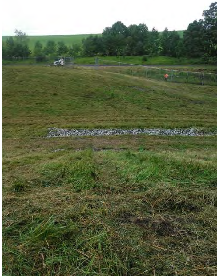
Photo 5 Mowed Vegetation & Drainage Structure (looking northwest)
