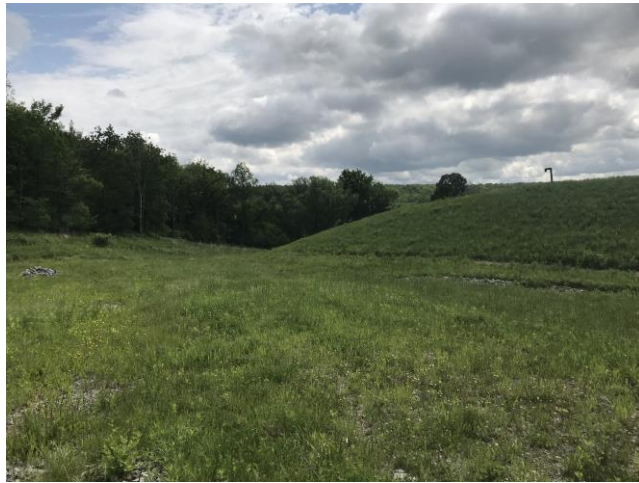
Northeast corner of the landfill
