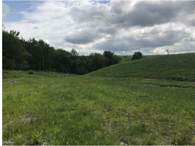
Northeast corner of the landfill
