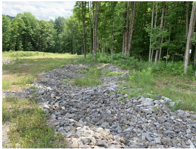
Drainage swale on the west side of the landfill.
