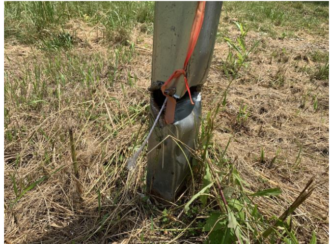
The casing associated with MW-2D has been damaged and the PVC riser has been clean cut. The riser is now approximately 1 foot above grade. Replacement of the casing and repair of the riser is necessary.
