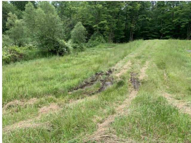
Ruts from lawn mowing operations noted between the landfill proper and the stormwater retention area to the south of the landfill.
