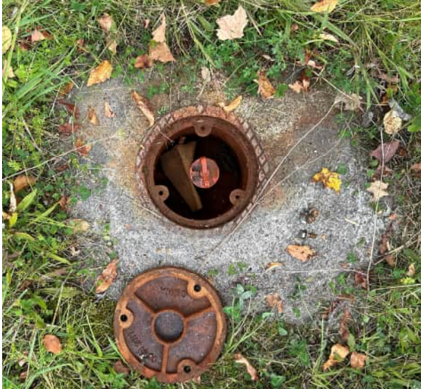
Rust coloring similar for MW-3BR2 and MW-3SR2.
