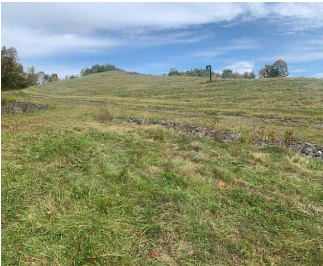
Southwestern side of the landfill. Landfill was recently mowed.
