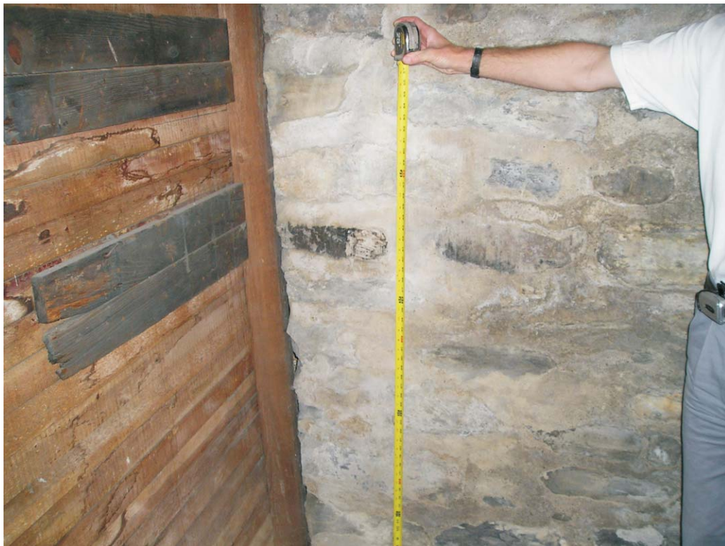
Photo #22: Stone #2 after sampling located approximately 3.5 feet above basement floor. Stone #3 is to the right of the measuring tape.
