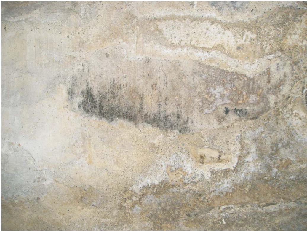
Photo #15: Stone #3 with mold or mildew appearance.
