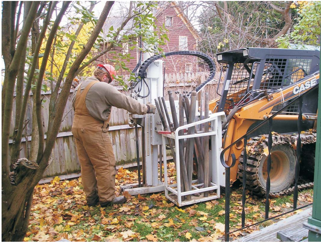
Photo #11: Skid steer mounted geoprobe unit advancing SB-07/PZ-02, looking east-southeast.
