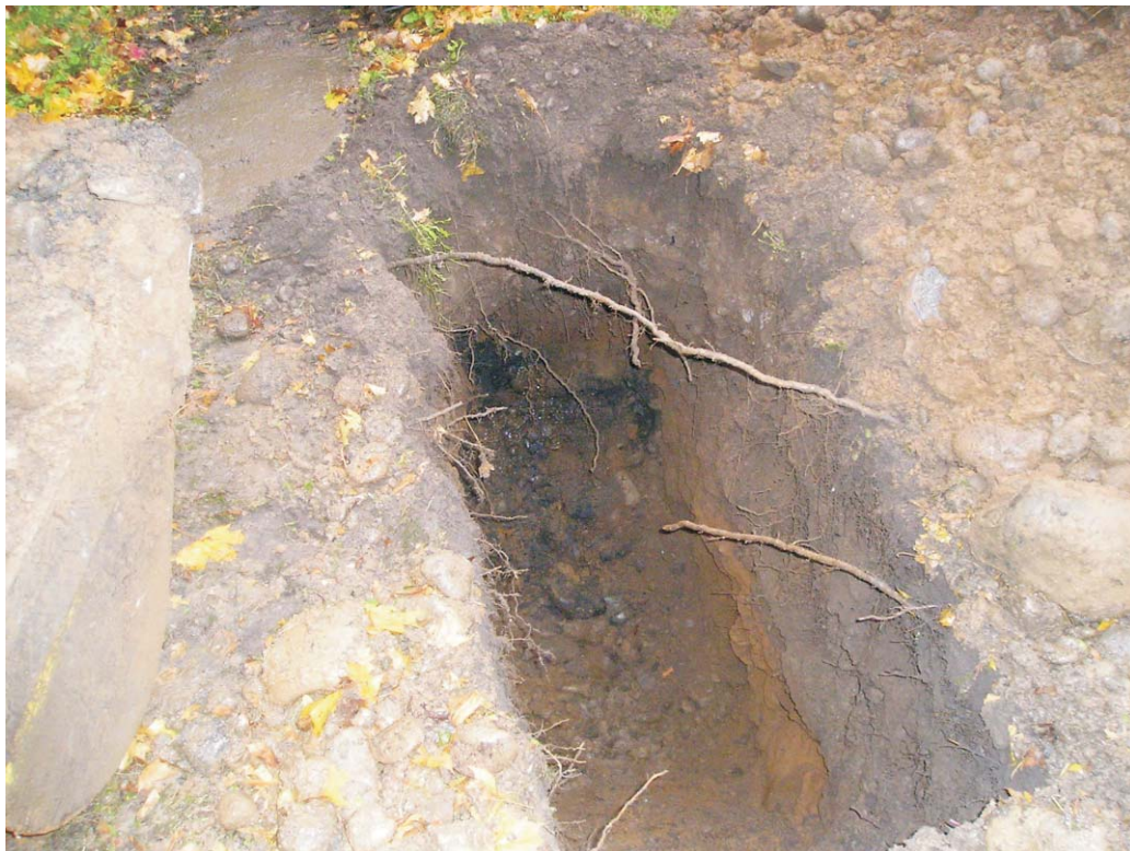
Photo #8: Test trench TP-02 excavated to approximately 7.0 feet below ground surface, looking north. Soils appear darker at north end of trench due to perched water percolating into trench.
