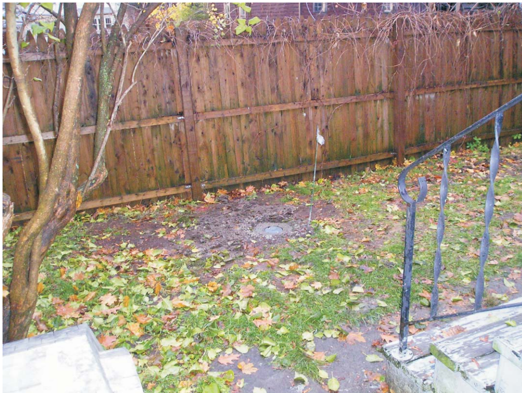
Photo #12: Surface completion at PZ-02.
