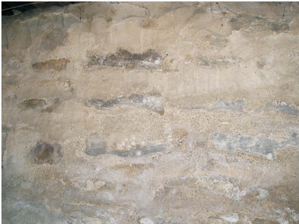
Photo #18: Background drill holes for collection of Scrape #3 sample, collected from the north wall.
