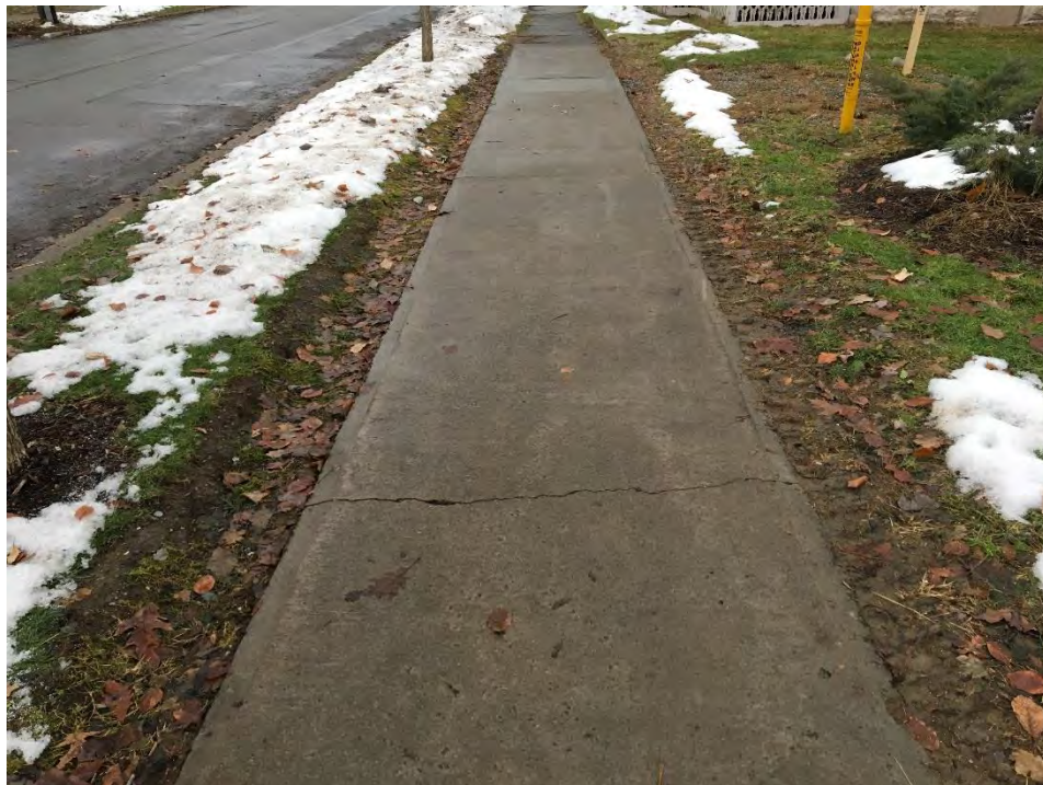
Photo 6: Crack observed in sidewalk, one of three on site, all located in line with curb side trees
