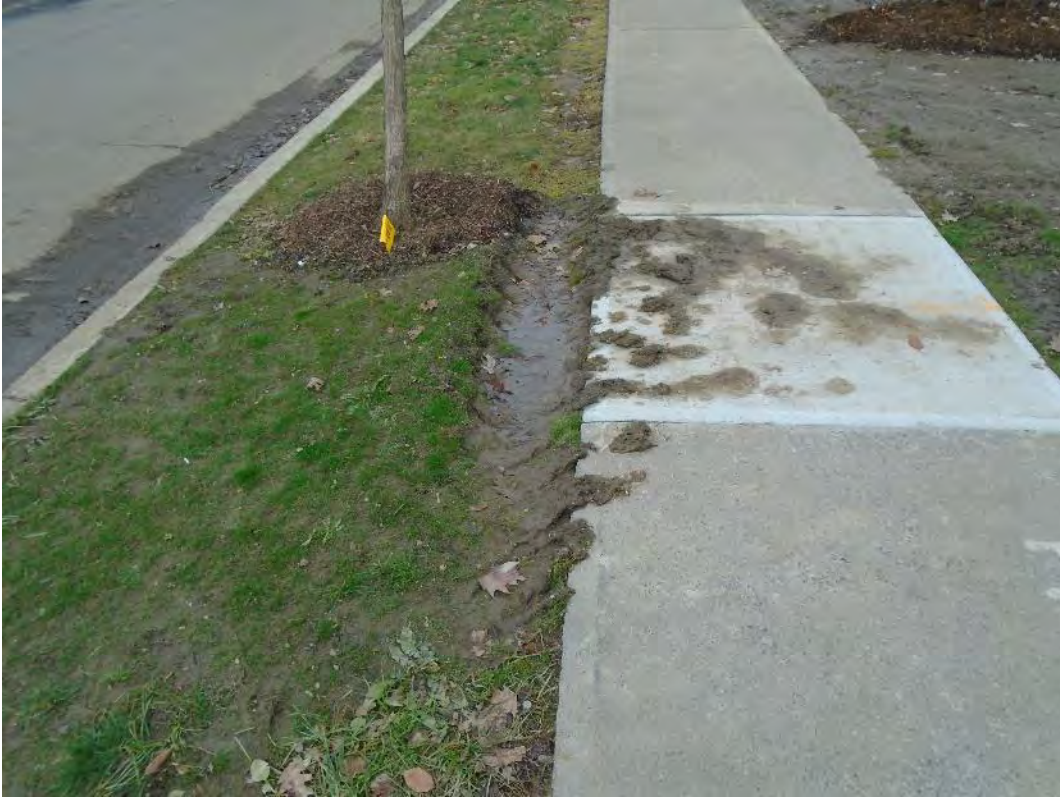
Photo 9: Ruts along sidewalk south end of site
