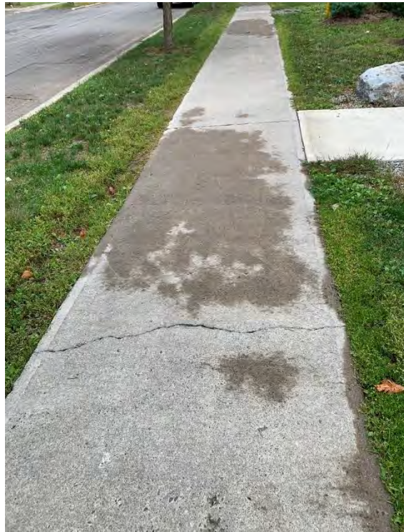
Photo 6: Crack observed in sidewalk, one of three on site, all located in line with curb side trees
