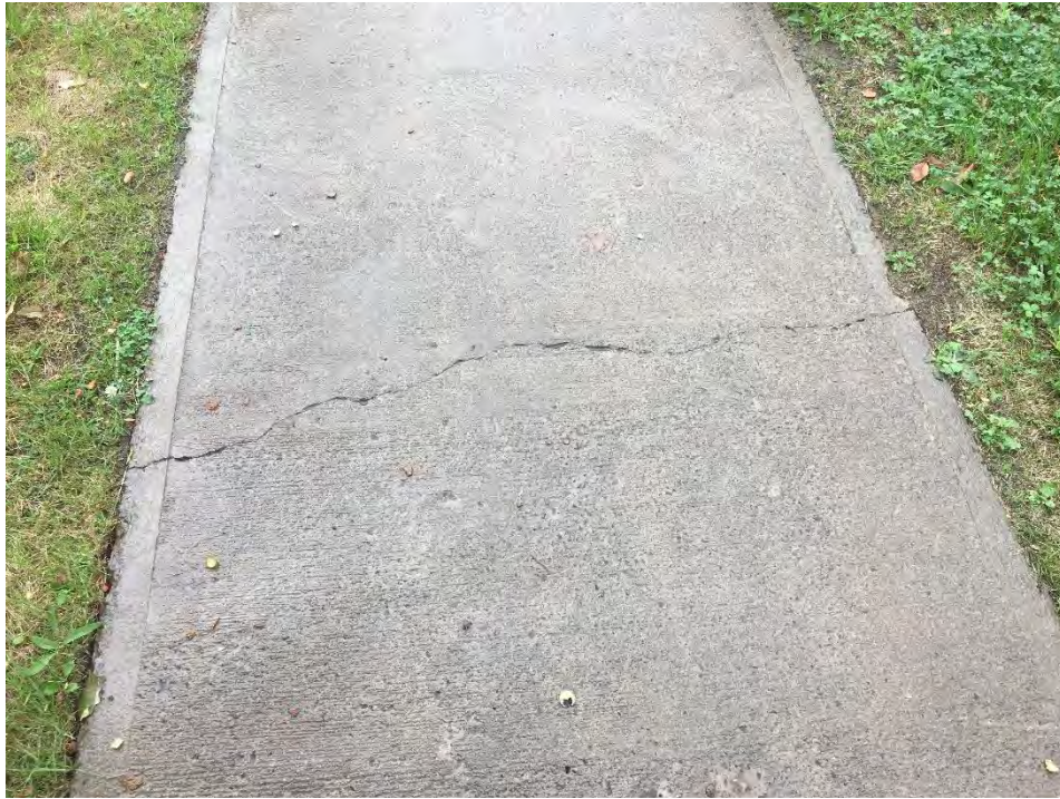
Photo 5: Crack observed in sidewalk, one of three on site, all located in line with curb side trees
