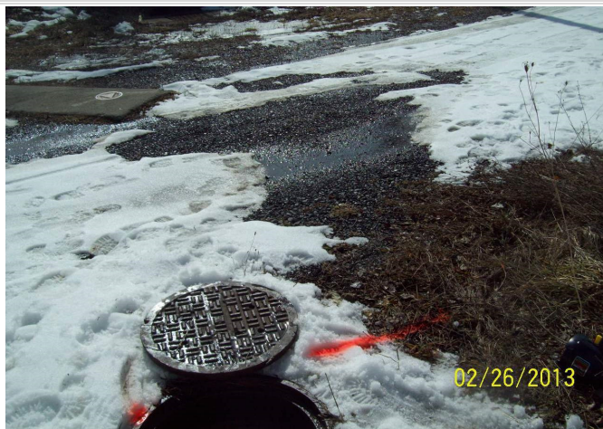
Photo 59 Unlabeled 24" diameter manhole near the vestibule on the south side of the Building.
