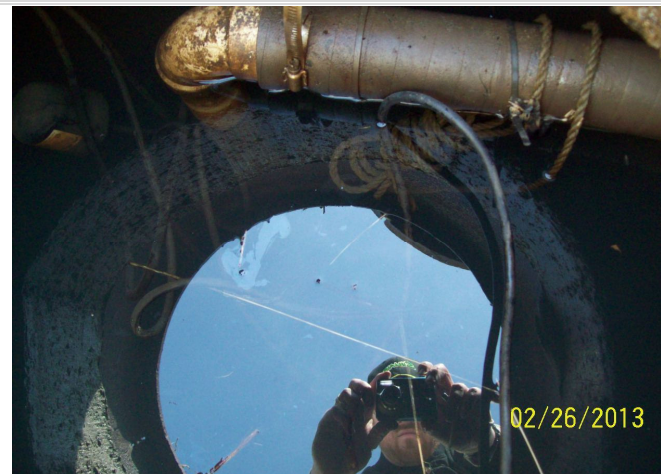
Photo 60 Unlabeled manhole interior containing standing water, an inoperable sump pump, and a 2-inch discharge pipe oriented toward the drainage ditch stormwater catch basin.
