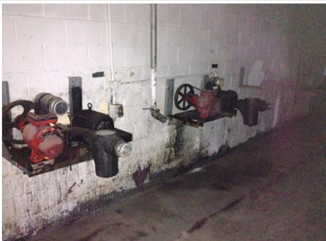
Photo 09 Transfer pumps mounted to wall in Tank Room.
