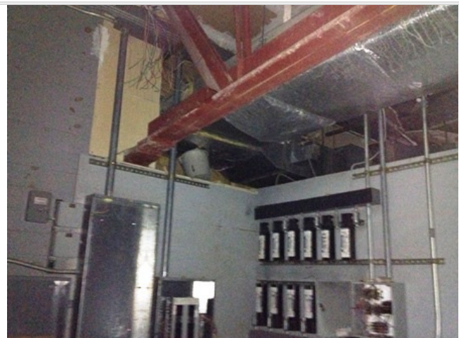
Photo 35 Electrical components on wall of Utility Room. Truss construction and partial insulation runs through the room and cut overhead wires remain in place.
