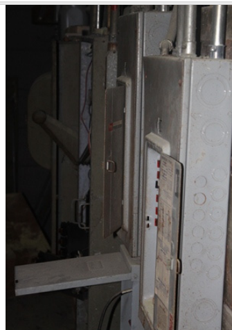
Photo 47 Left: Front entrance boarded, broken glass remains. Right: Electrical panels on the exterior wall of wood frame of building near the Conference Room. Electrical boards contain asbestos.
