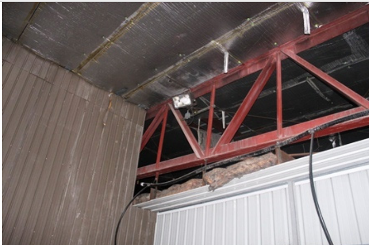
Photo 27 Overhead steel truss supporting new metal building structure.
