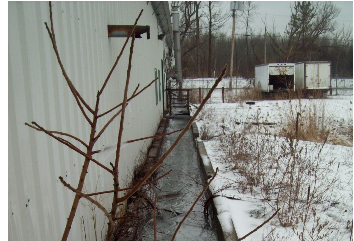
Photo 50 Stormwater collection trench located along the west side of the building looking south.
