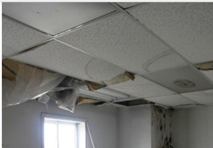
Photo 31 Office in southwest corner of building; deteriorating roof.
