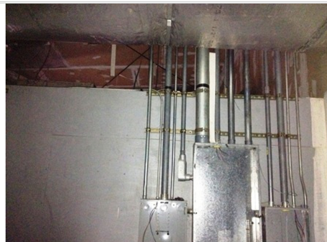
Photo 36 Utility Room. Electrical panels on wall and raceways out of the room.
