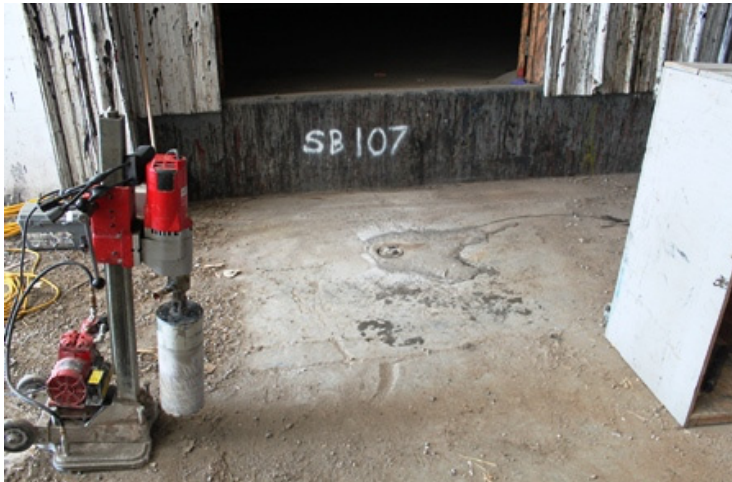
Photo 17 Step up into Lab Pack Staging and Consolidation Area No. 1 from unloading area (approximately 30" in height). Concrete core on the left shows the floor slab thickness in the unloading area.
