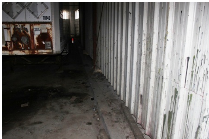
Photo 05 Stained concrete floor slab in Truck Unloading Pad Area.
