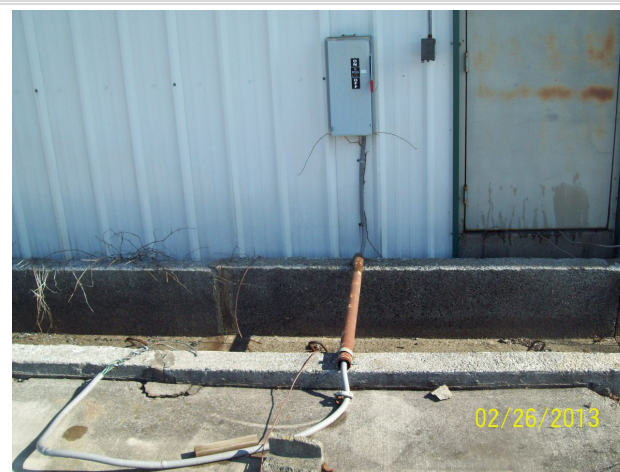
Photo 56 Existing out-of-service electrical box and conduit on the west side of the building.
