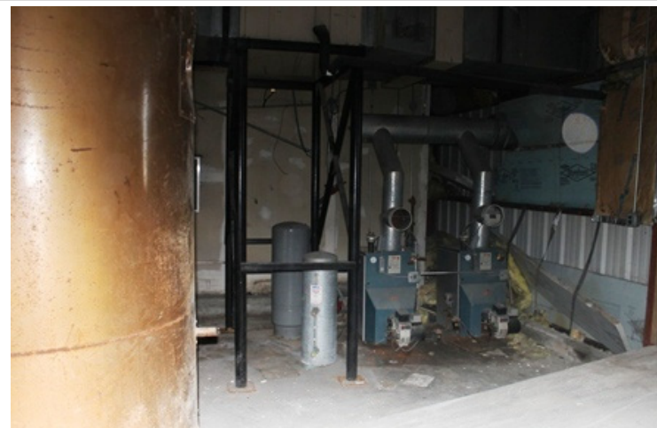
Photo 30 Boiler Room concrete slab elevation lower than entrance. Fuel oil-fired building heating system. The fuel oil tank was previously removed.
