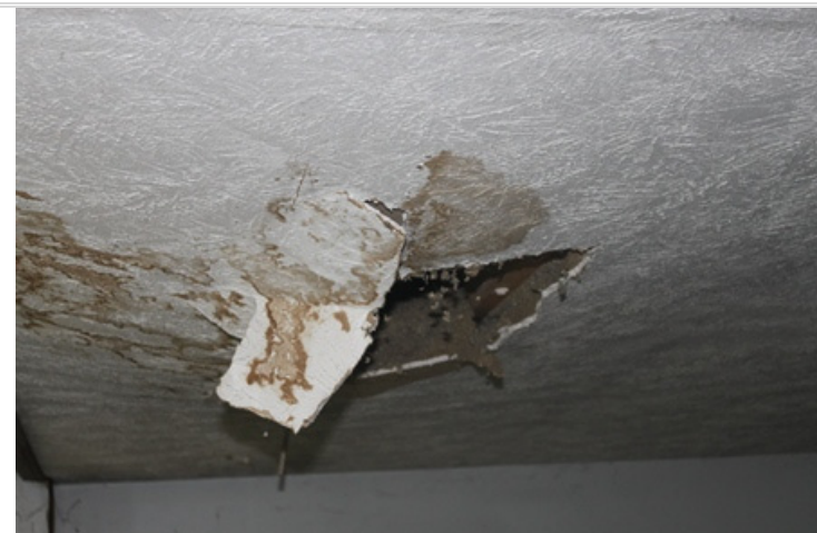
Photo 44 Office in southwest corner with ceiling deterioration.
