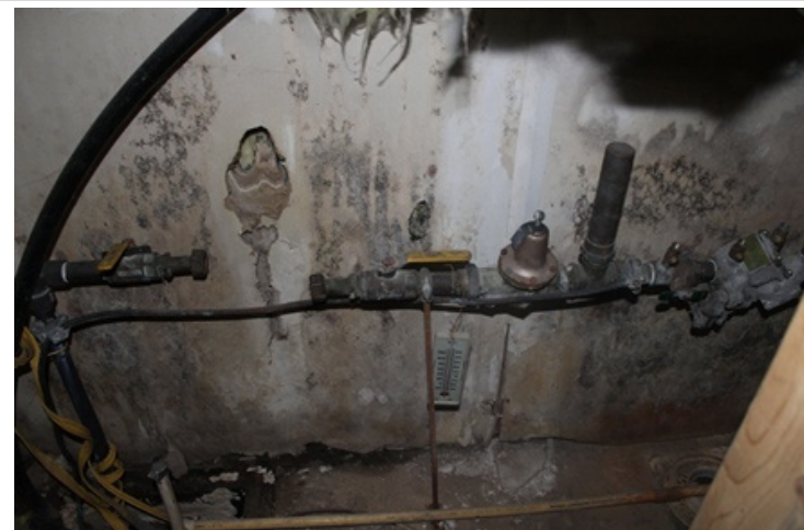
Photo 34 Utility Room water service connection with evidence of mold.
