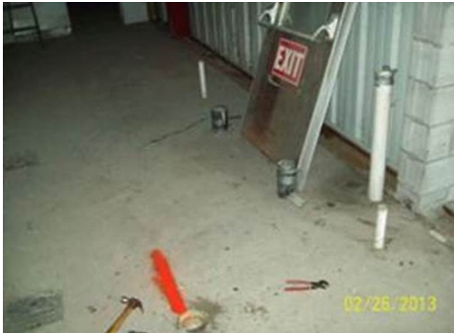
Photo 49 Four aboveground pipes co-located with a sanitary cleanout within the main entrance vestibule area of the building.
