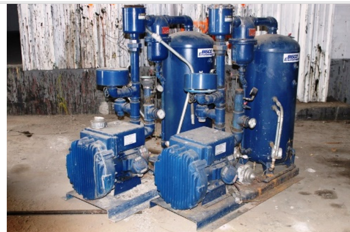
Photo 24 Skid mounted soil-vapor extraction (SVE) systems. Each SVE system includes a Rotron Model EN858BD72WL blower and Solberg Model No. CSL-851-250HC vacuum filter.
