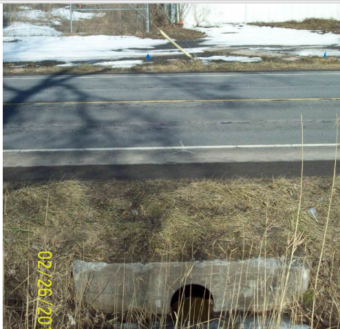
Photo 51 Culvert that conveys stormwater from the drainage ditch along Canal Road to the Site looking north.
