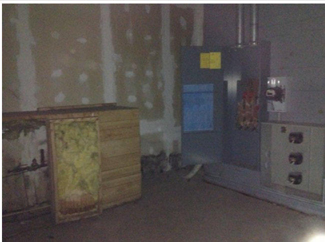
Photo 33 Utility Room near southwest corner of building. The electrical panels have been partially dismantled.
