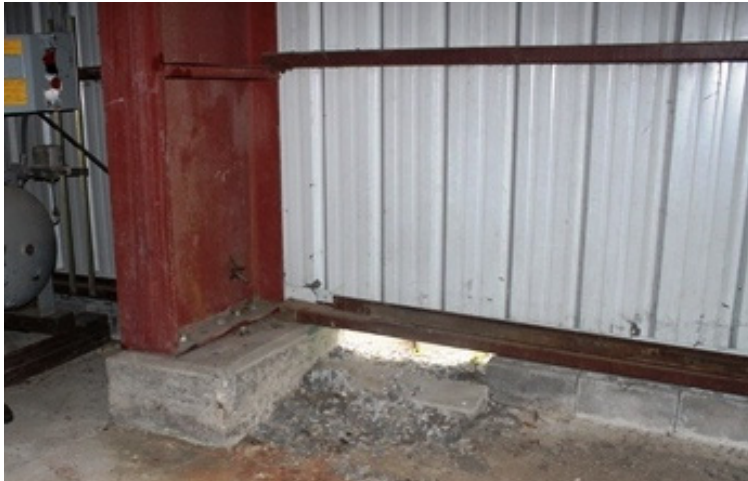
Photo 25 Concrete footing and pre-fabricated metal wall. The wall does not extend to the ground surface. Therefore, the building is not fully enclosed.
