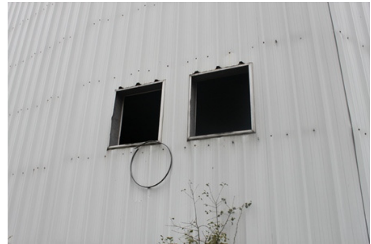
Photo 02 Exposed windows with no glass or pane located on eastern wall of building.
