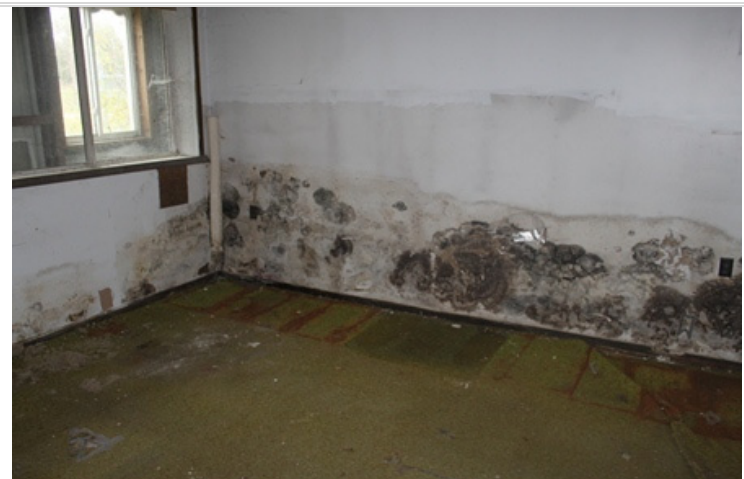
Photo 43 Office in southwest corner with mold on wall.
