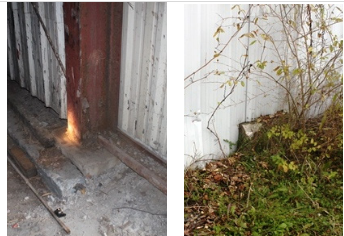
Photo 04 Concrete block that serves as column support on east side of building. Left: Photo shows inside metal building wall. Right: Shows concrete block protruding outside of metal building wall.
