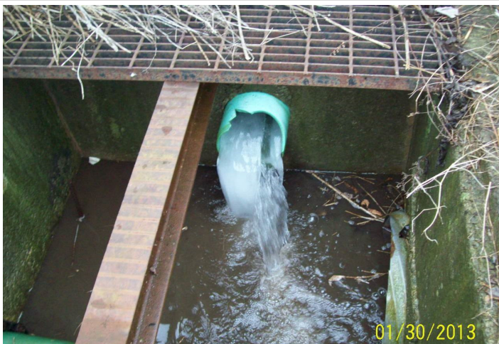
Photo 53 Catch basin next to the stormwater collection trench. This catch basin receives discharge from the stormwater collection trench and the catch basin to the south.
