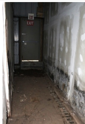
Photo 38 Left: Overhead construction near Laboratory and Office Supplies Room. Right: Exit to southwest side of building (apparent mold at the base of drywall).
