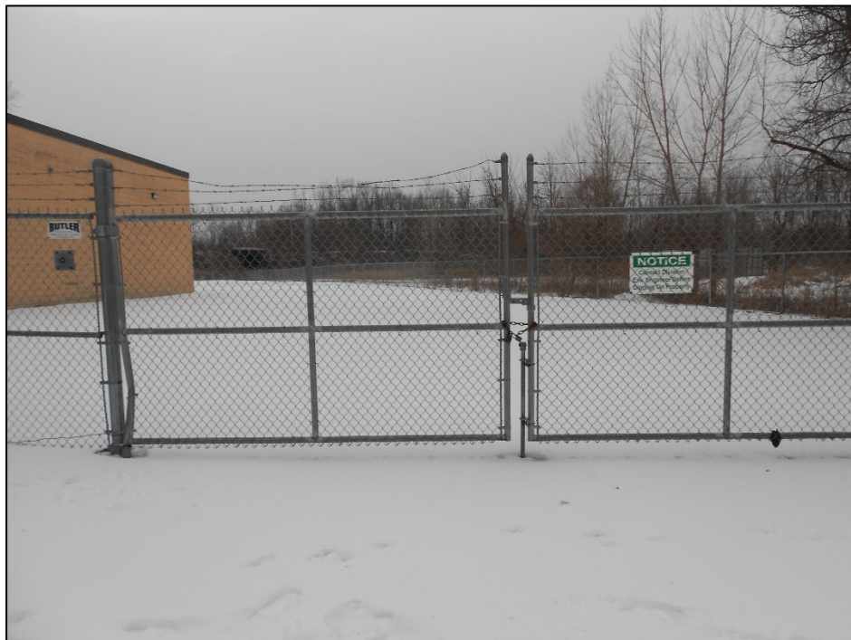
January 13, 2022 – Site Conditions
