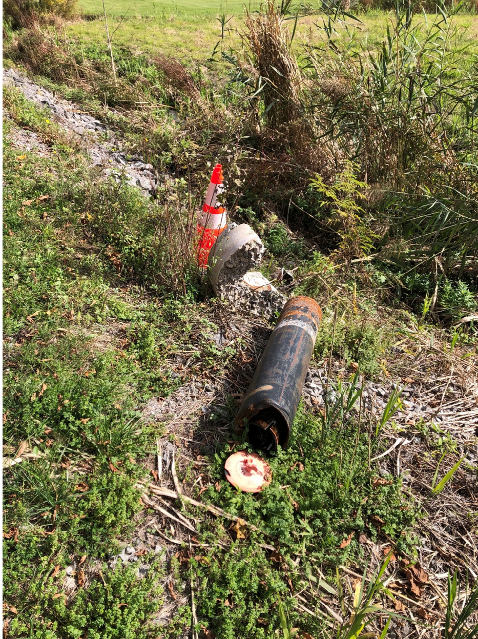
October 12, 2022 – RW-1 condition
