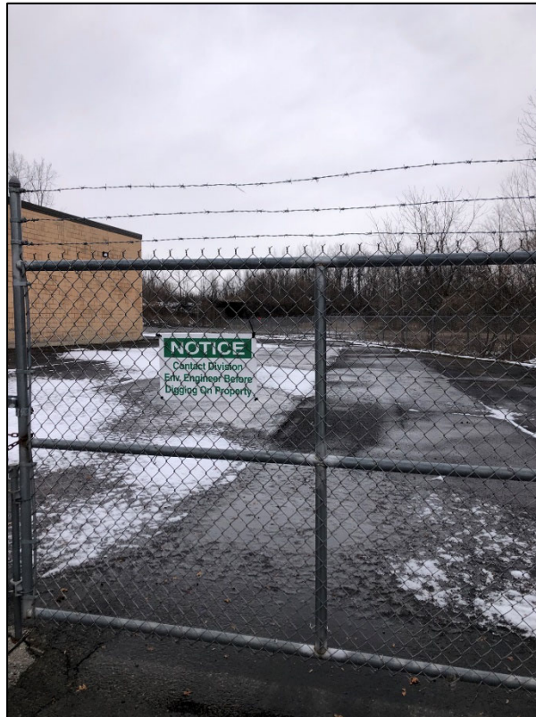
January 11, 2024– Site Conditions
