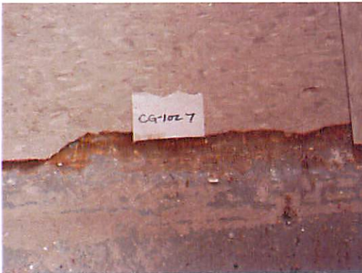
12" X 12" Floor Tile and Mastic
