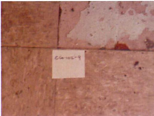
12" X 12" Floor Tile and Mastic
