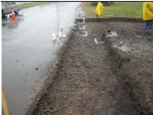
Picture 1: Sidewalk excavation and bollard layout
