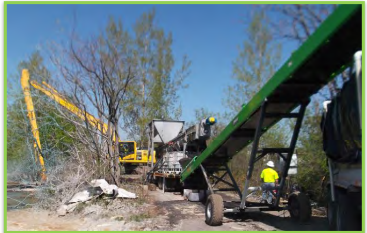
Figure ES-4: Semet Residue Removal Dewatering and Conveyance Field Demonstration
