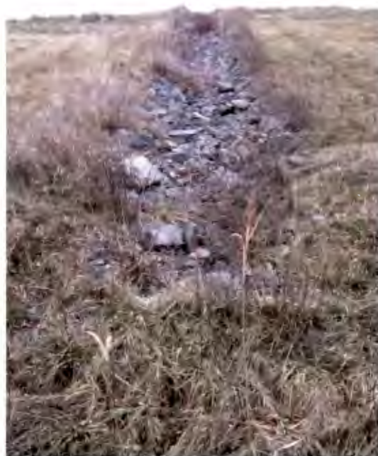
Figure 6 Drainage ditch on side slope.
