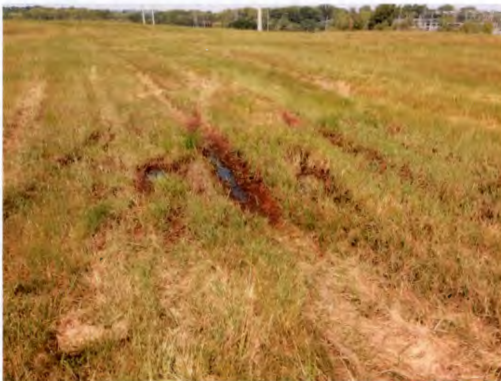
Figure 7. Ponded water near gas vent on top of landfill. July 2015.
