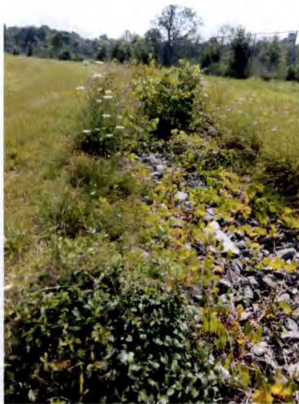
Figure 8. Small trees and tall plants grwoing through rip-rap in drainage ditch near SW corner of landfill. July 2015
