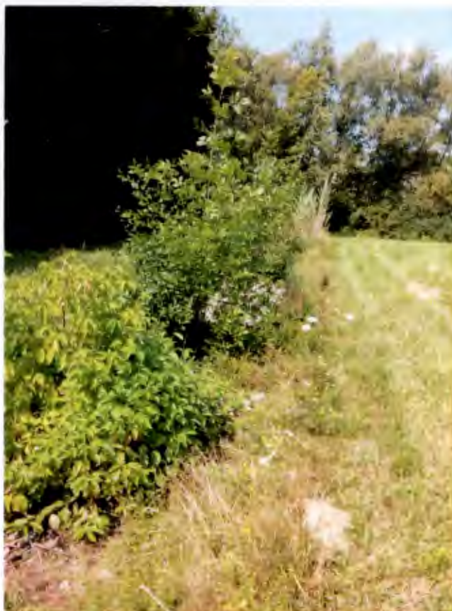
Figure 9. Small trees and tall plants growing through rip-rap in drainage ditch near SW corner of landfill. July 2015
