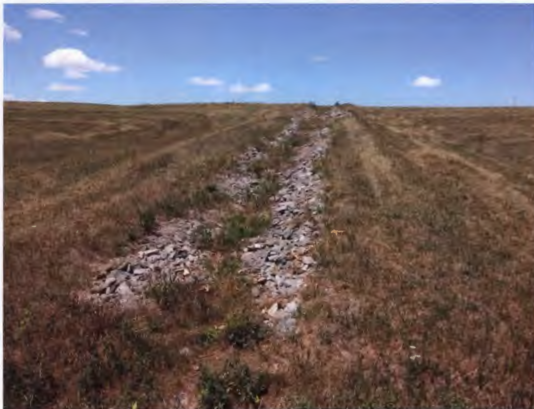
Photo 7. Drainage down chute in good condition without woody plants – August 2016.
