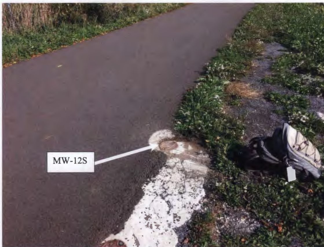
Photo 10. Monitoring wells MW-12D (bottom of photo) and MW-12S after removing blacktop to re-gain access for groundwater sampling – October 2016.
