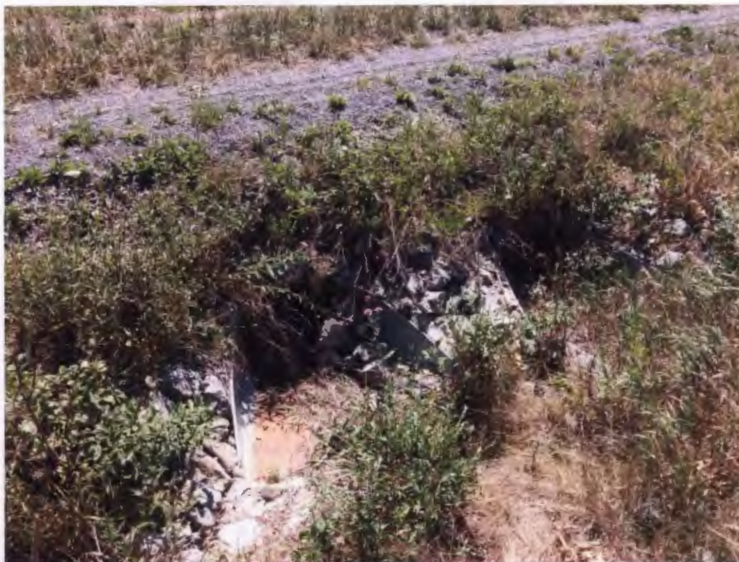
Photo 8. Culverts under access road. Generally clear with slight plant overgrowth – August 2016.
