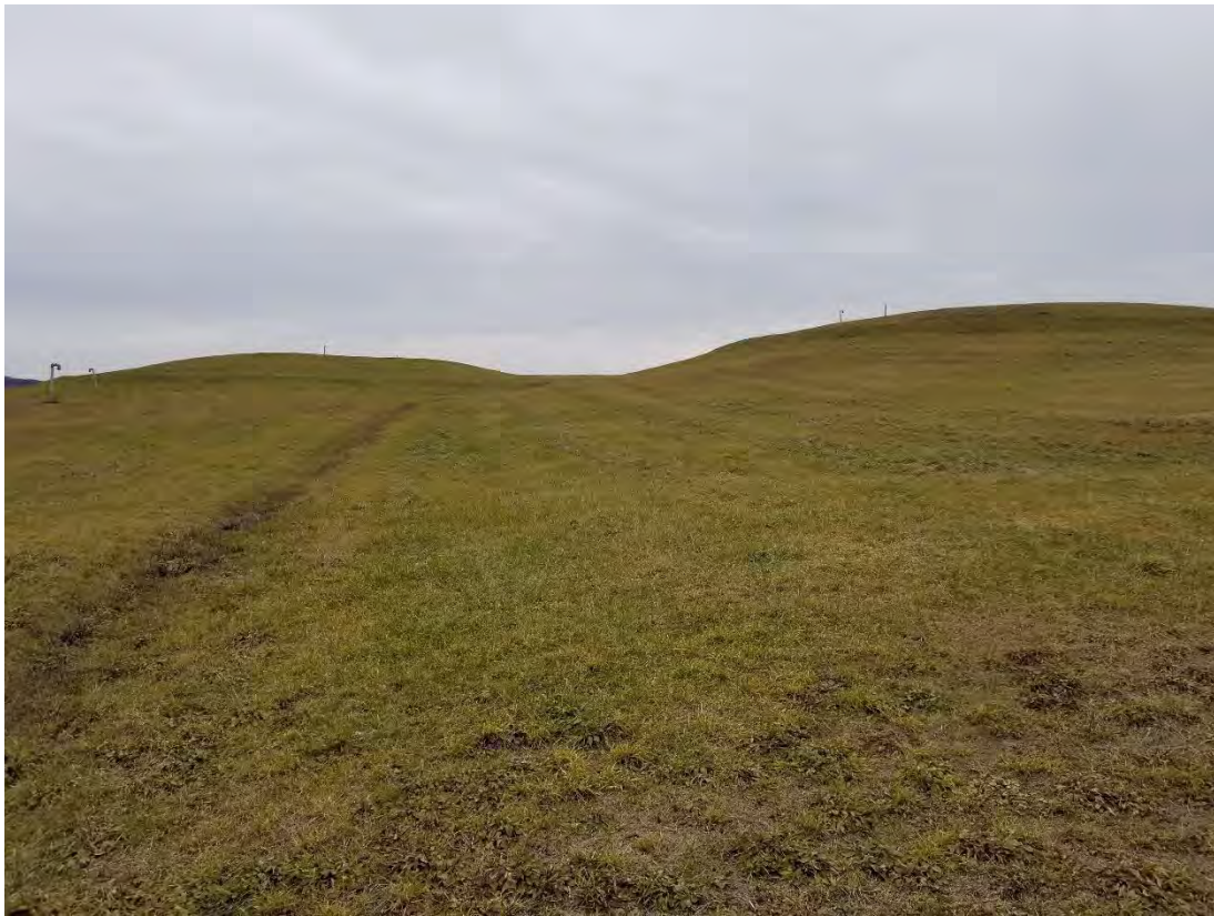
Photo 7. Mowed grass and gas vents in distance. – December 2017.
