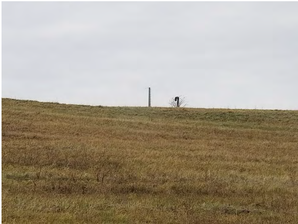
Photo 6. Gas vent with small tree growing out of reach of mower. – December 2017.
