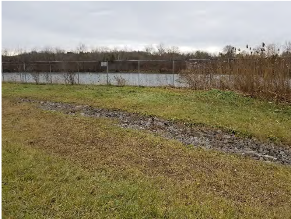
Photo 5. Maintained down chute viewing North at Erie Canal. – December 2017.
