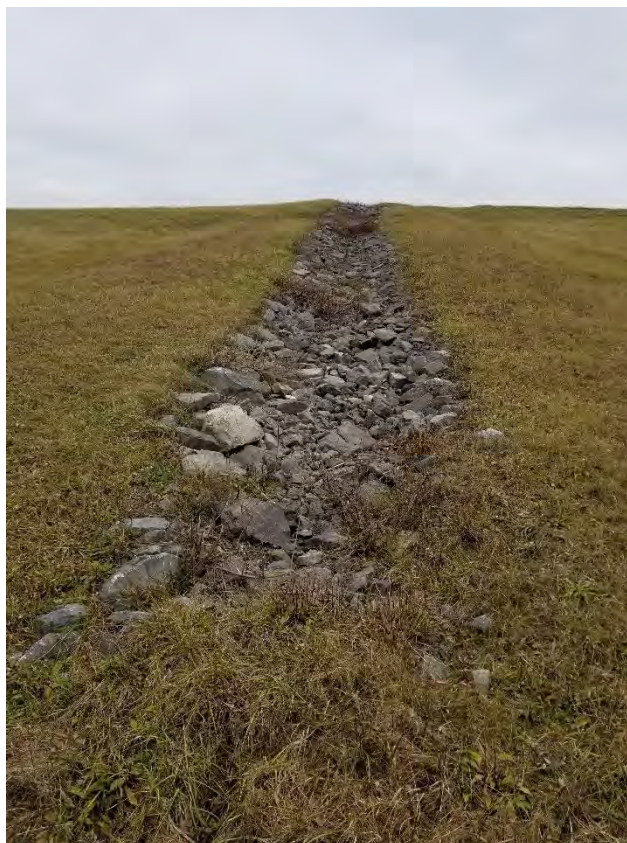
Photo 2. Drainage down chute in good condition without woody plants – December 2017.
