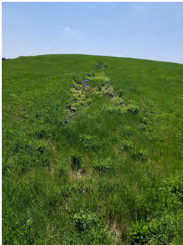
Photo 2. Drainage down chute in good condition without woody plants – May 2018.
