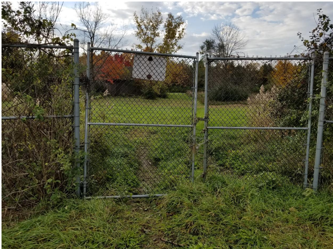
Photo 8. Access gate at SE corner of landfill near canal barn at Cedar Bay. – October 2018.
