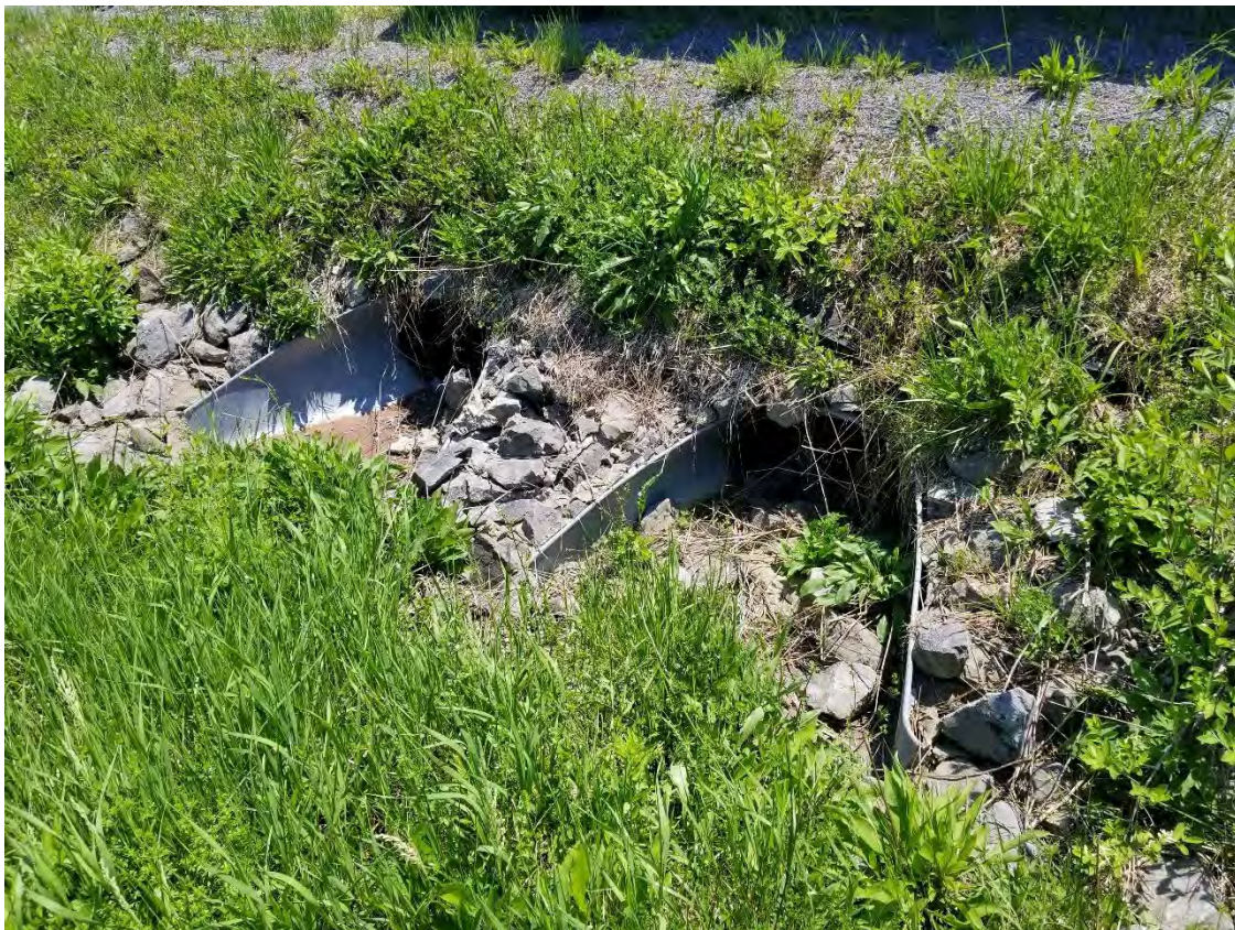
Photo 10. Dual storm water culverts under access road. – May 2018.
