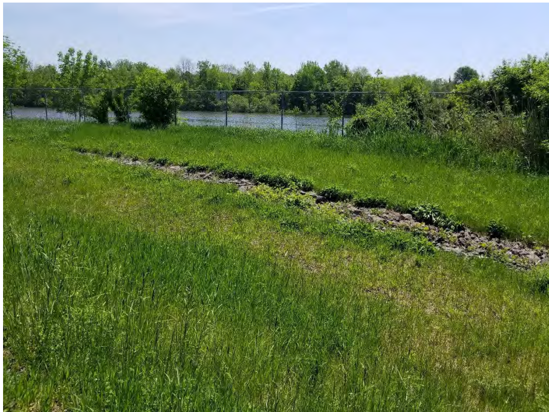
Photo 4. Down chute with small trees removed since 2016. – May 2018.
