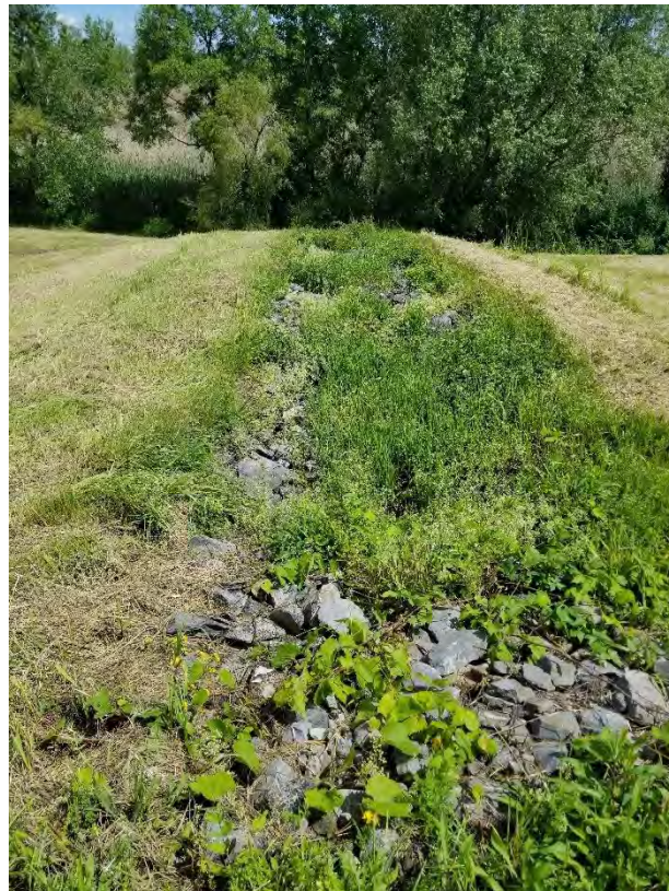
Photo 2. Drainage down chute in good condition without woody plants – June 2019.
