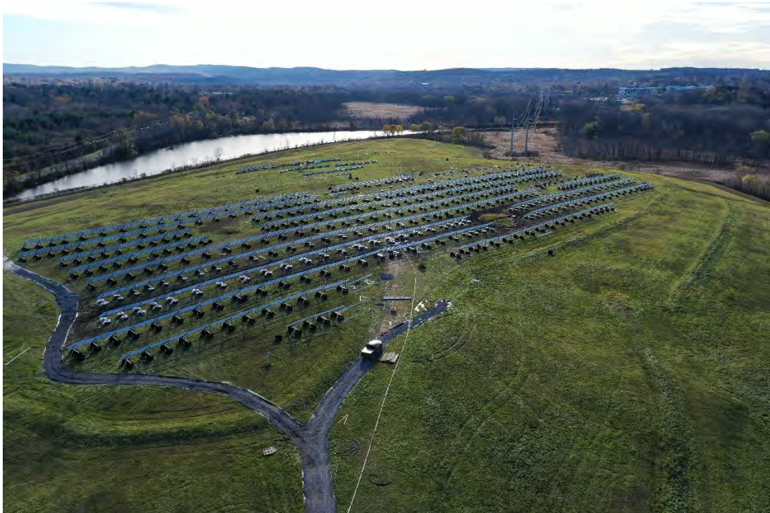
Photo 10. Viewing southwest at partial construction of solar panel frames and concrete pad pumping operation. - November 2019.
