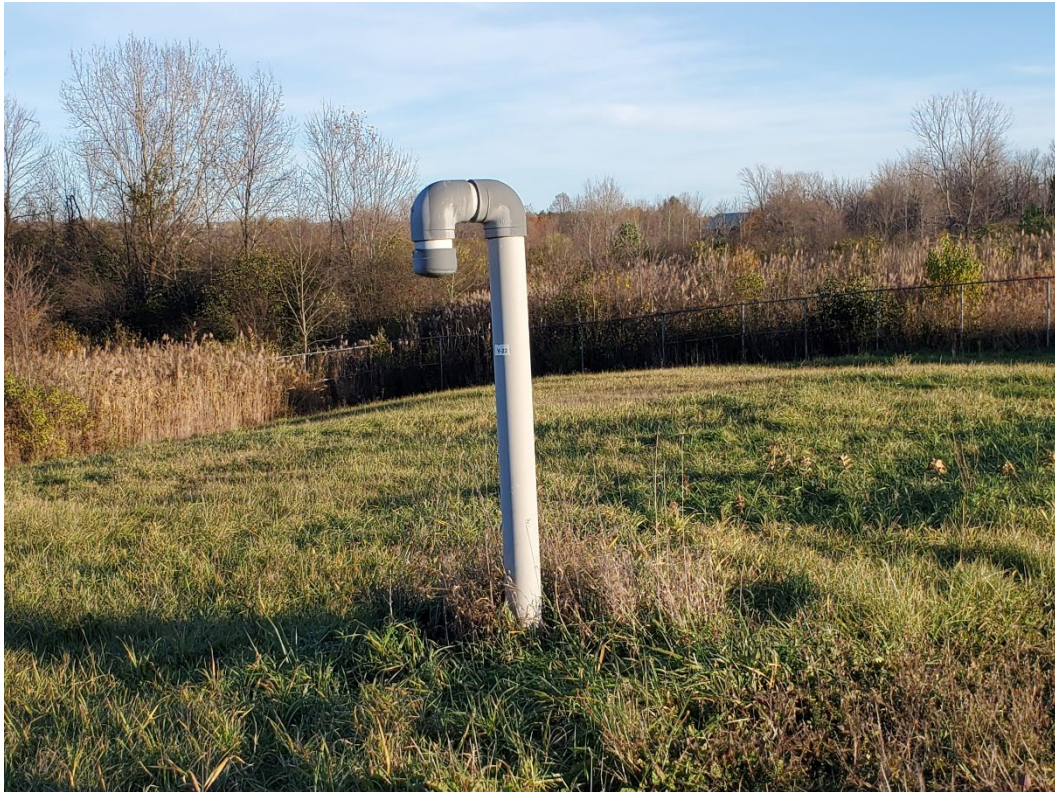
Photo 3. Gas vent V-22 clear of woody growth. – November 2021.
