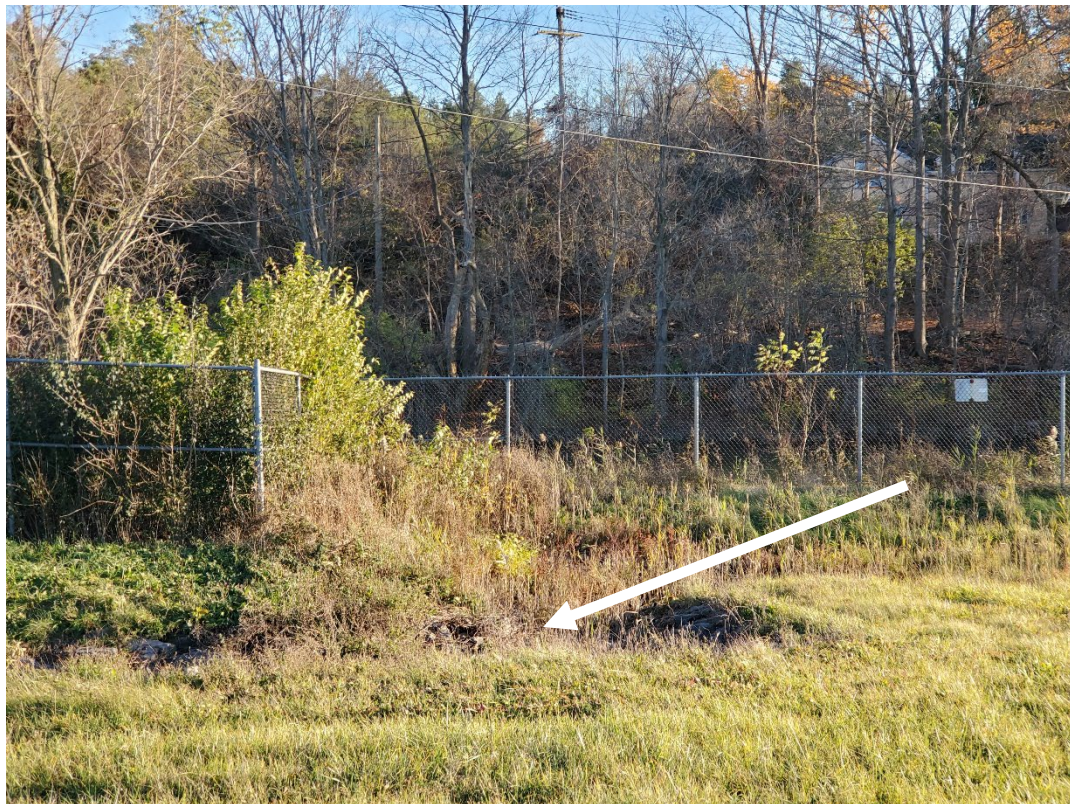
Photo 4. Surface run-off collection swale on south perimeter, viewing south toward canal. November 2021.
