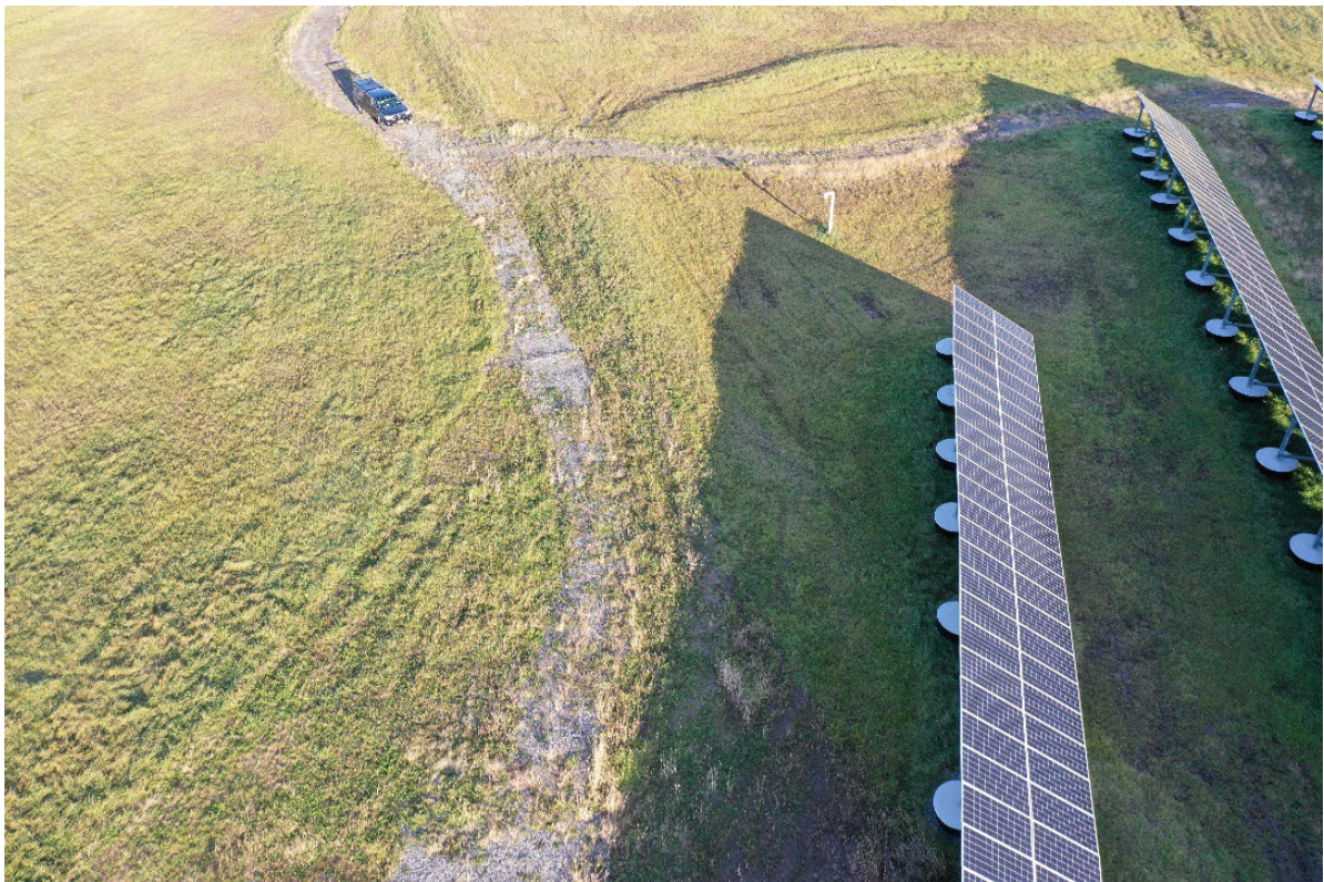
Photo 8. Viewing east at top of landfill and back side of solar array – November 2021.
