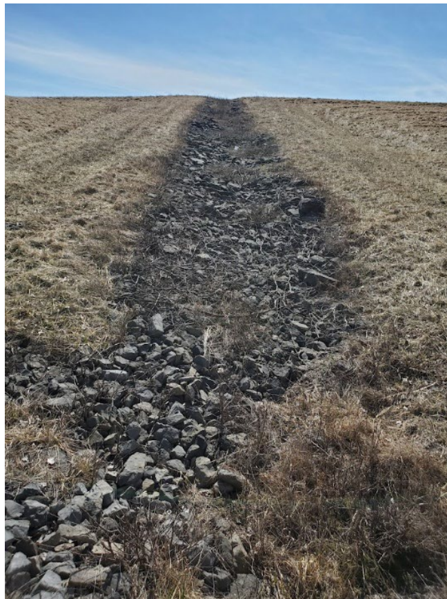
Photo 6. Down chute on NW corner of landfill is open and clear. – March 2024.
