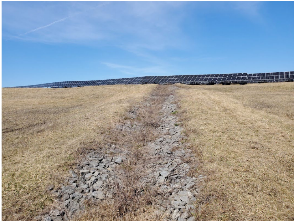
Photo 8. Viewing north at top of landfill and front side of solar array. – March 2024.
