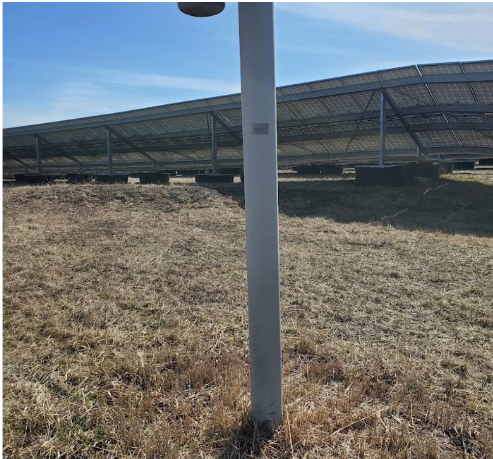
Photo 3. Typical Gas vent. – March 2024.
