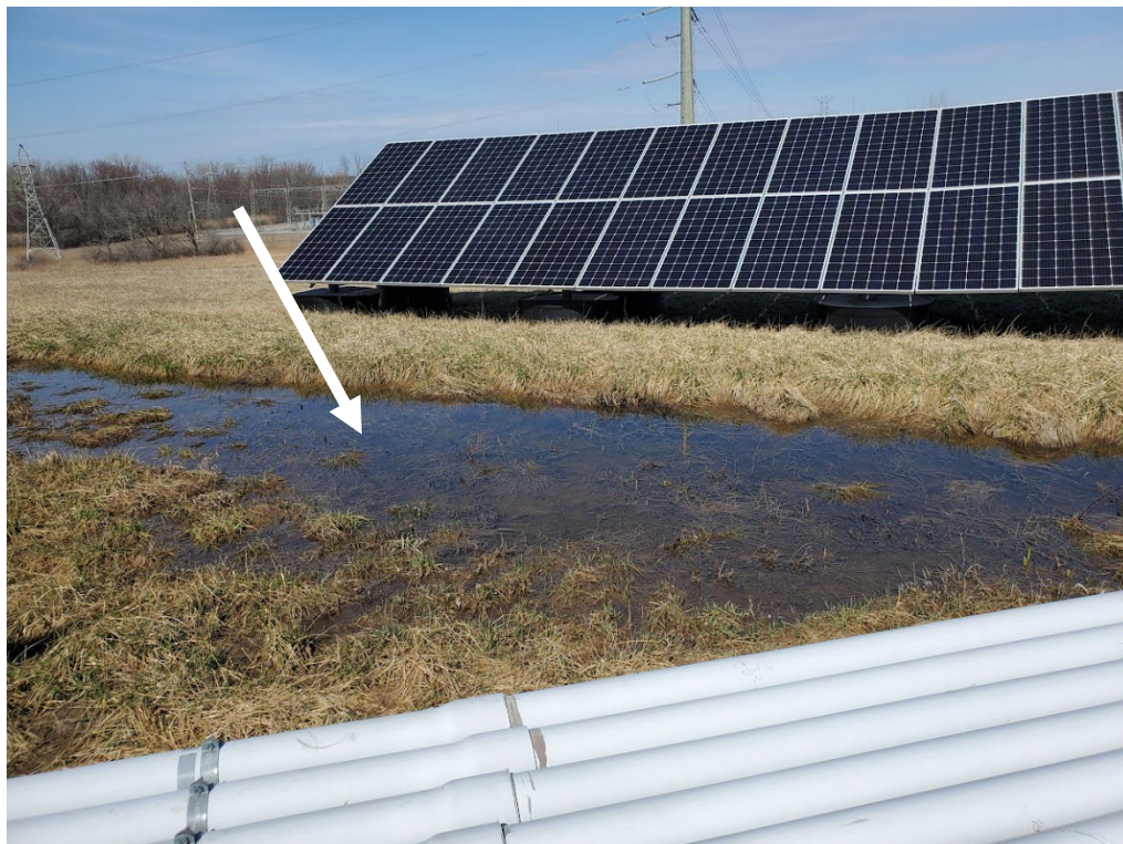
Photo 4. Temporary wet spot from spring rains and snowmelt, viewing northeast toward solar panels. March 2024.
