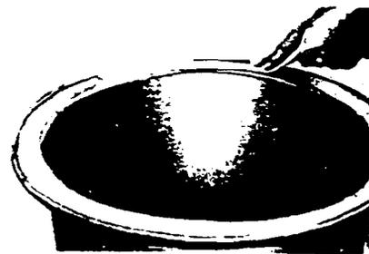
Fit basin cover over discharge pipe. Power cords are sealed with split rubber stopper. Rubber ring is placed over discharge pipe and compressed between pipe and cover by the flange (chamfered side down) form a seal. Thread vent pipe into flange on basin cover.
