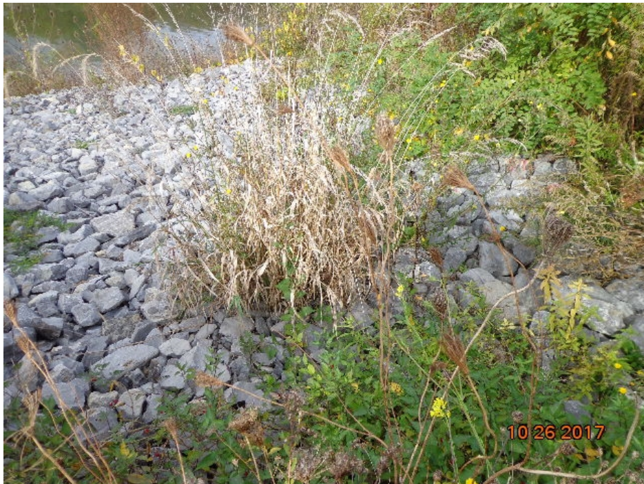
Photograph Number 10: Stormwater outfall rip-rap area leading to Nine Mile Creek.
