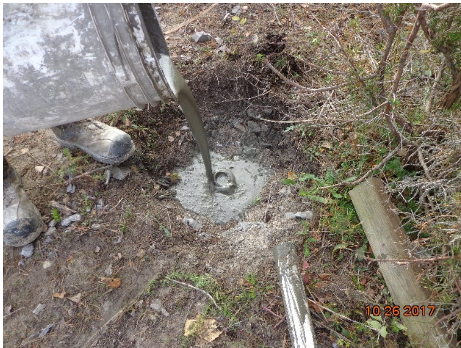
Photograph Number 14: The steel protective casing was removed and the PVC casing was cut down to 1-foot below ground surface. Remainder of void was backfilled with bentonite grout and bagged topsoil.
