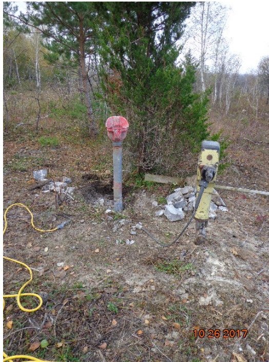
Photograph Number 13: A bentonite grout mixture was placed in the PVC casing using a tremie rod.
