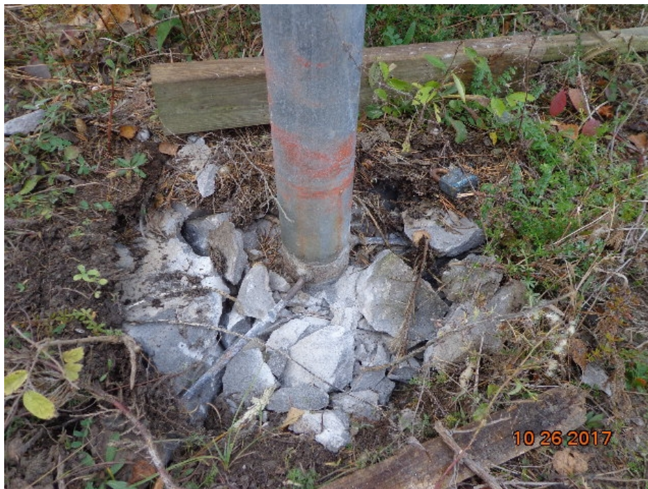
Photograph Number 12: The concrete pad was broken away and removed.
