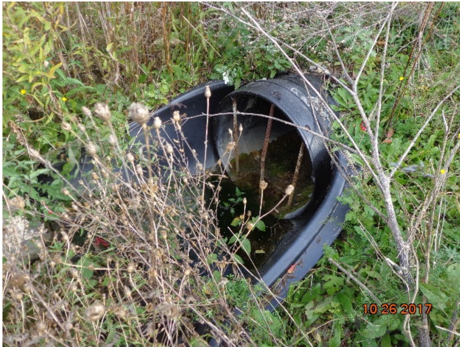
Photograph Number 9: Stormwater outfall pipe.
