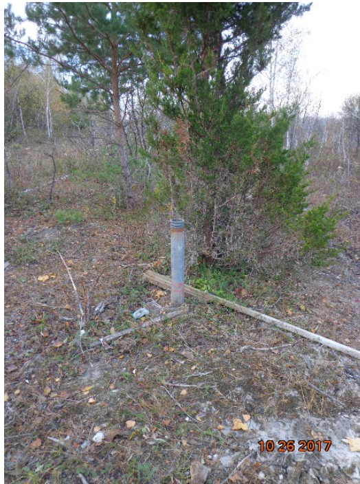
Photograph Number 11: Monitoring well W-5.5 prior to decommissioning.
