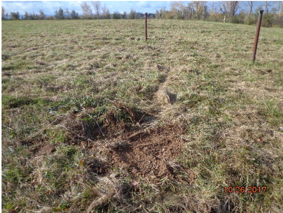
Photograph Number 15: MS-106.5 following decommissioning. Well was decommissioned in same manner as W-5.5.
