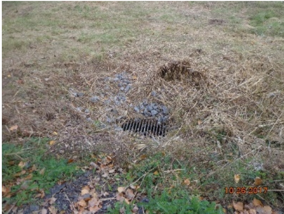
Photograph Number 5: Representative view of stormwater catch basin after annual mowing.
