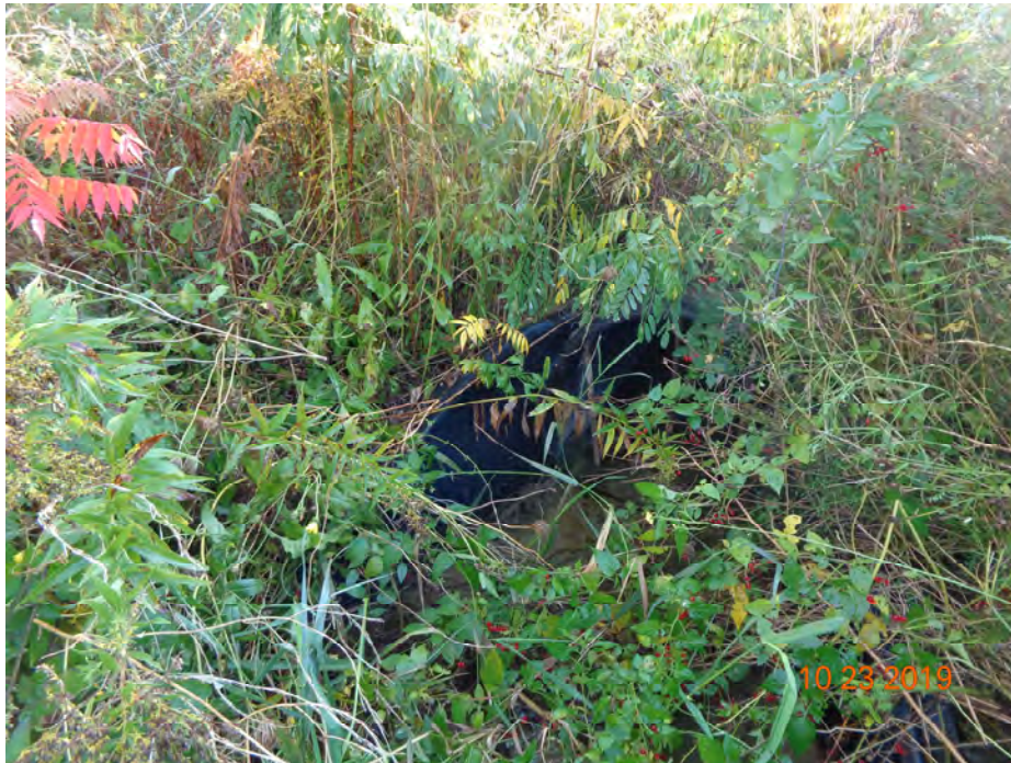
Photograph Number 8: Stormwater outfall pipe.
