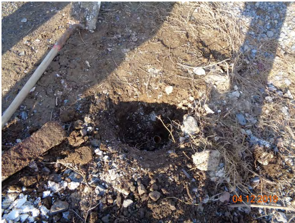
Photograph Number 12: DW-103 after decommissioning. The well screen and casing was filled with bentonite grout, the steel protective casing was removed and the PVC casing was cut down to 1-foot below ground surface.
