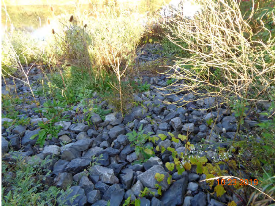
Photograph Number 9: Stormwater outfall rip-rap area leading to Nine Mile Creek.
