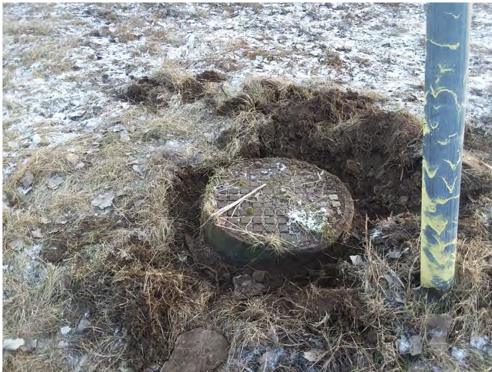
Photograph Number 16: View of repositioned manhole MH-4 cover. The dug out soil and sod was replaced around the manhole cover.
