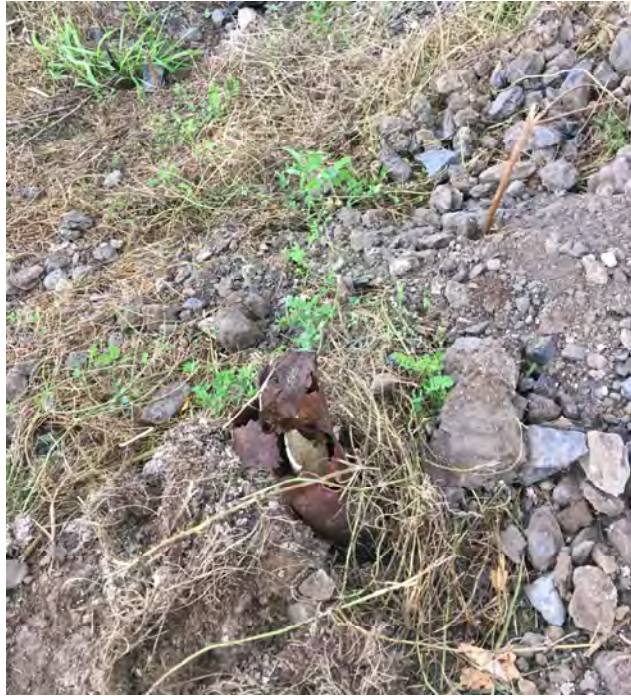
Photograph Number 11: Monitoring well DW-103 prior to decommissioning.
