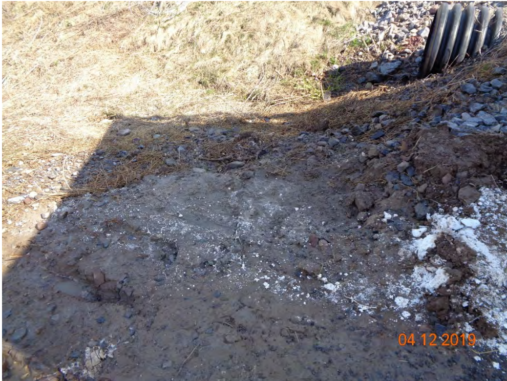
Photograph Number 13: The DW-103 decommissioning surface void was backfilled with bentonite grout and bagged topsoil to match surrounding grades.
