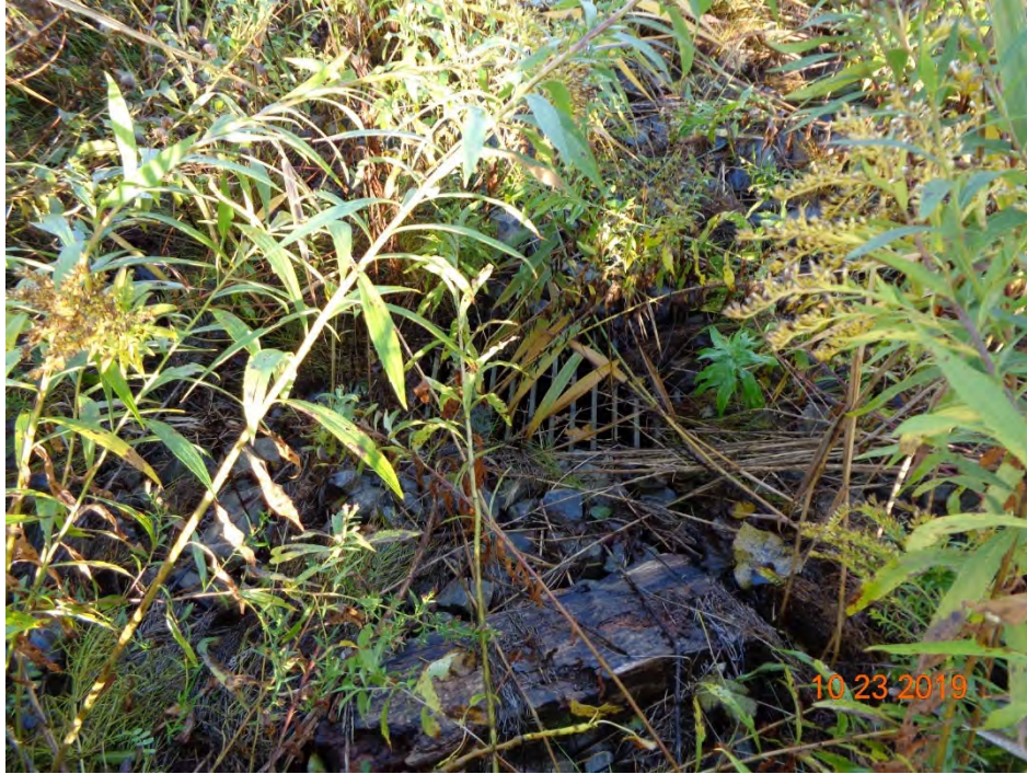
Photograph Number 5: Representative view of stormwater catch basin
