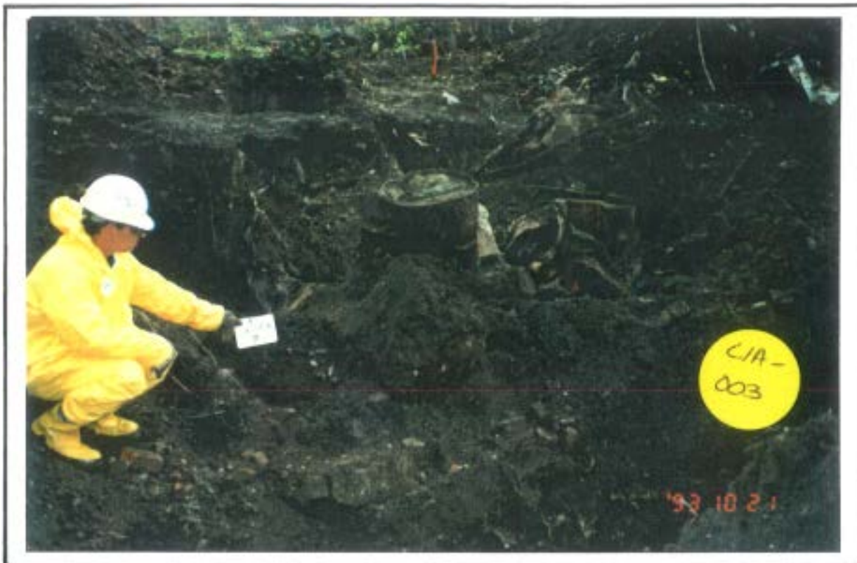
Photograph 7 - Test Pit CIA-003 - Partially Uncovered Drums
