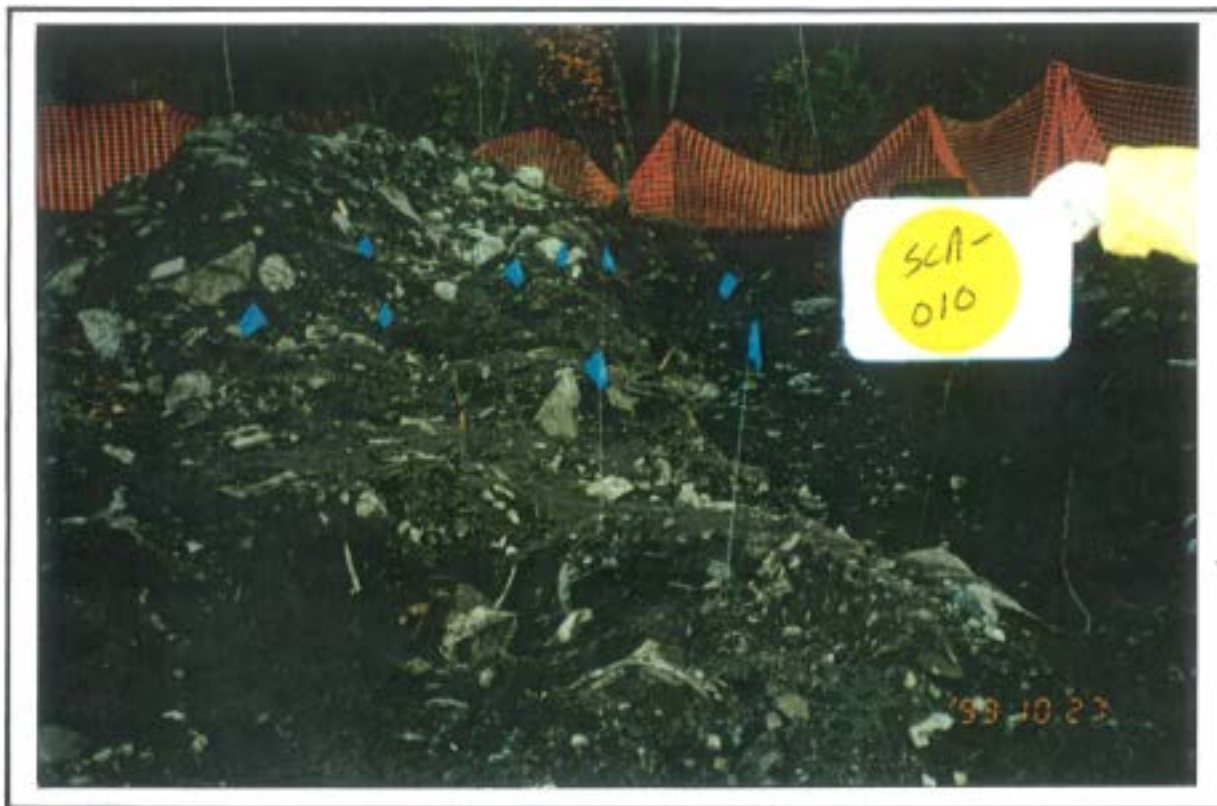
Photograph 3 - Test Pit SCA-010 - Blue Flags Locate Individual Drums Partially Uncovered
