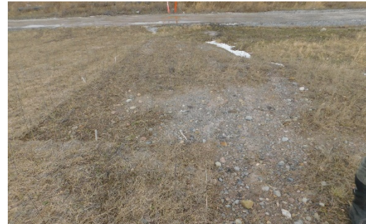
Minor erosion rills forming at toe of previously installed RECP
