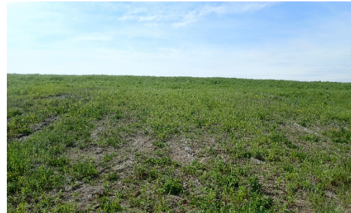
Minor erosion rills noted at toe of RECIP at the northern edge of the site
