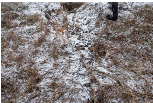
Erosion rill noted on western slope
