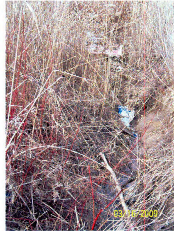
87 Drainage from culvert crossing Thompson Road
