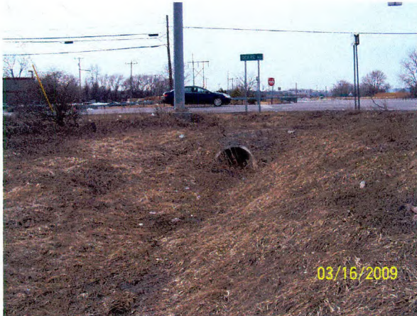
81 Culvert at Deer Road looking west
