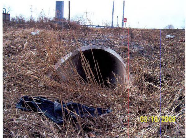
82 Culvert at Deer Road looking west
