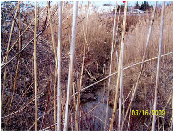
92 North drainage to culvert area
