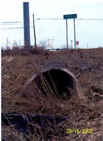
83 Culvert at Deer Road looking west
