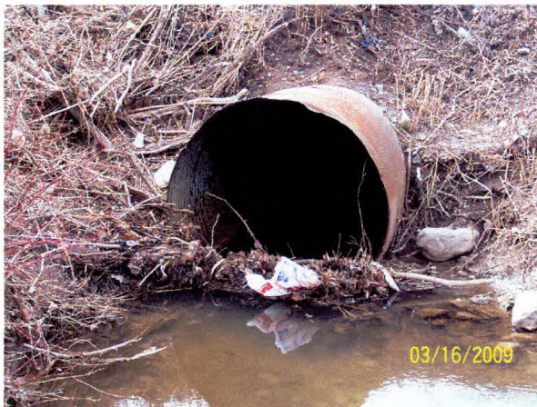
90 Culvert at Mautz Road looking west
