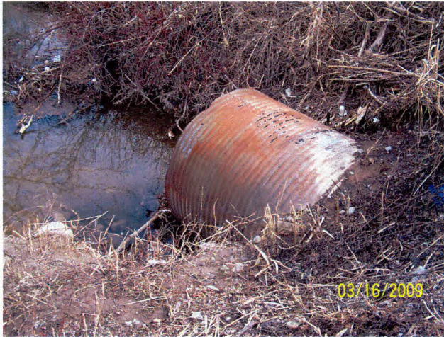
86 Culvert at Mautz Road looking east from North; ~ 18 inch diameter
