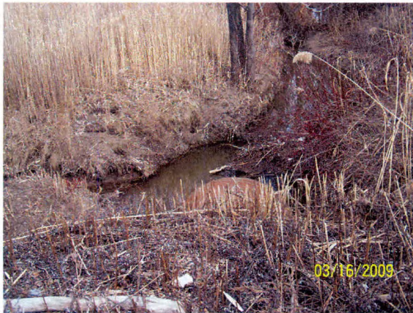
95 Culvert at Mautz Road looking east
