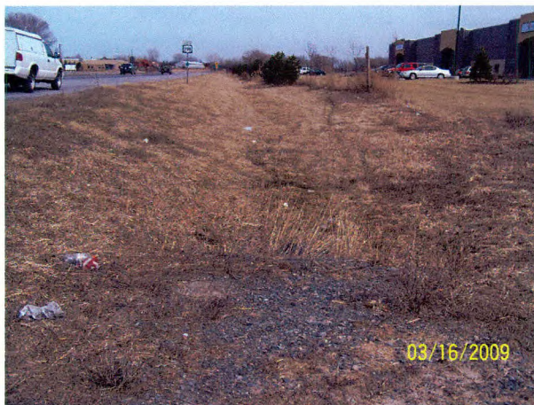
85 Drainage ditch leading to Deer Road culvert
