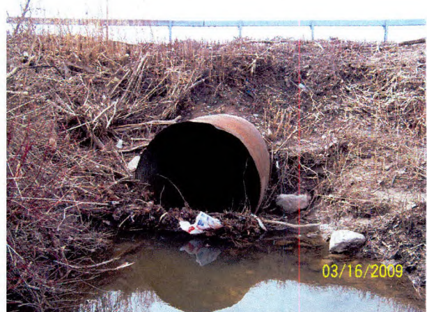
91 Culvert at Mautz Road looking west
