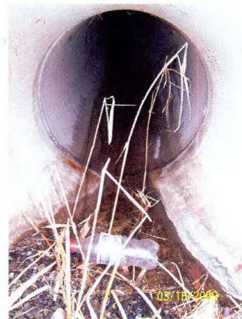
84 Culvert at Deer Road; about 18 inch culvert
