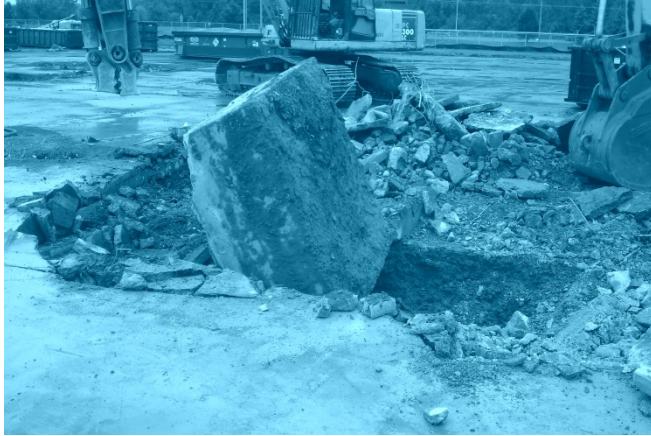
Photo 1: Interim Action Photo, Substation I
