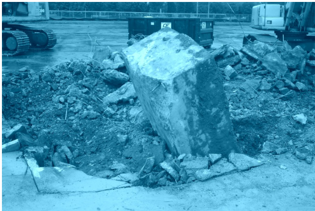
Photo 3: Interim Action Photo, Substation I
