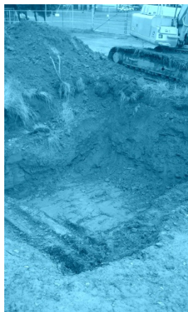
Photo 5: Interim Action Photo, Substation I
