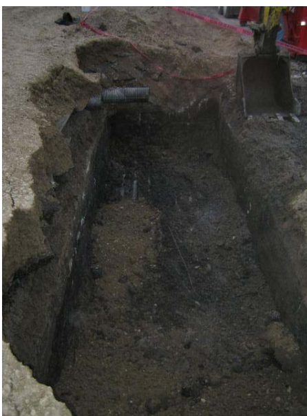
View of the vault and backfill materials – October 2011.
