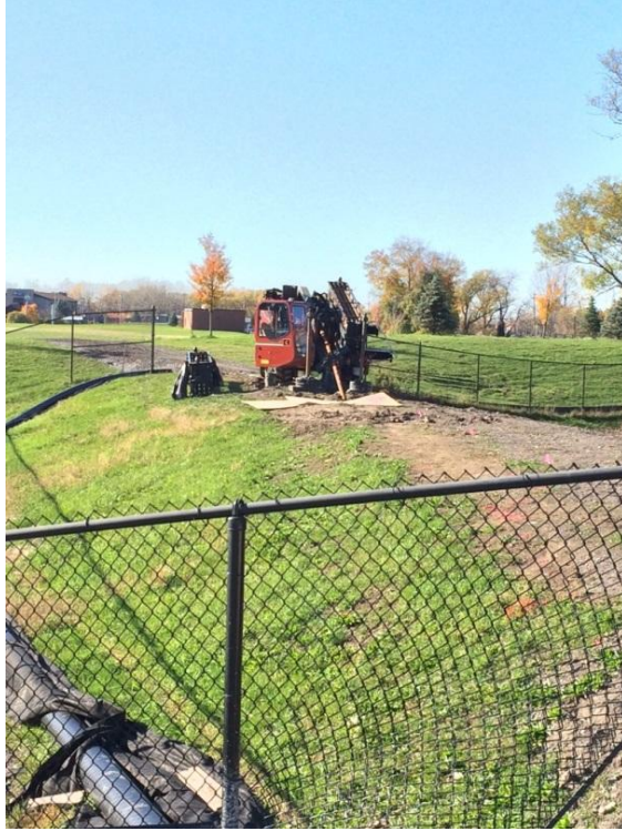
Entrance for Directional Drilling of Horizontal Well (West End)
