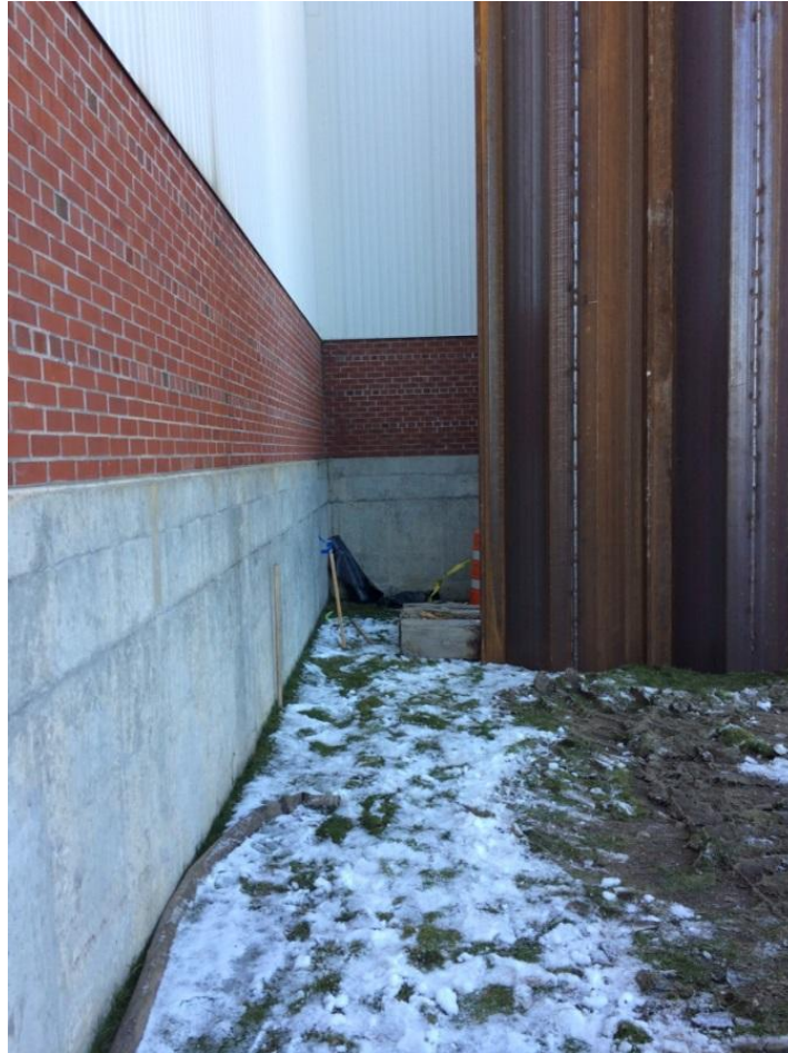
Sheet Return Wall at East End
