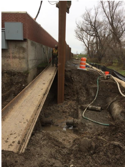
Installation of Sheetting – East end of TR-3 North Wall
