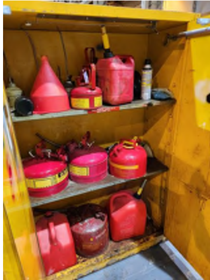
Photo Title: 20221221_161026.jpg Date: 12/21/2022 Description: Flammable storage cabinet in TR-5 warehouse area.
