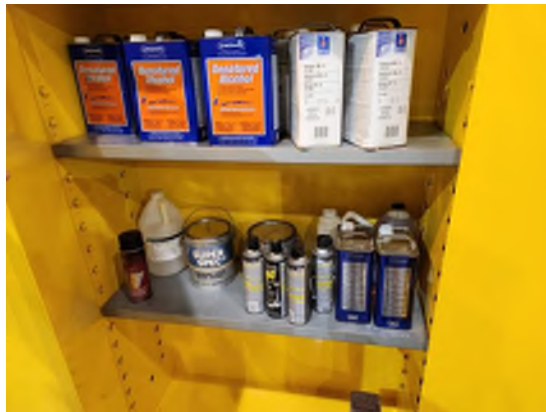
Photo Title: 20221221_160809.jpg Date: 12/21/2022 Description: Flammable storage cabinet in TR-5 warehouse area.
