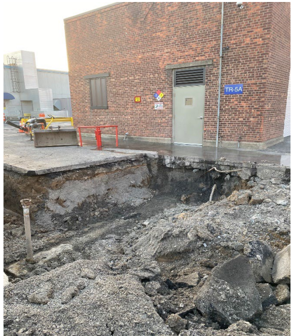
4 - PROXIMITY TO BUILDING WALL IMG_6054
