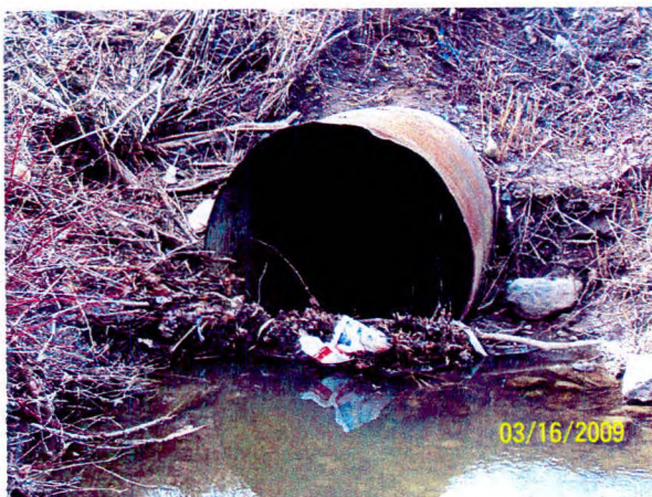
90 Culvert at Mautz Road looking west
