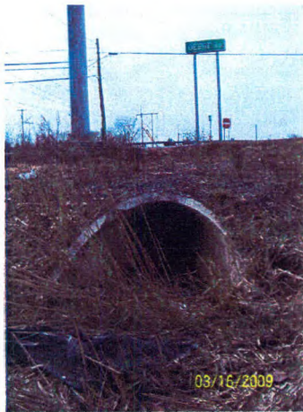
83 Culvert at Deer Road looking west
