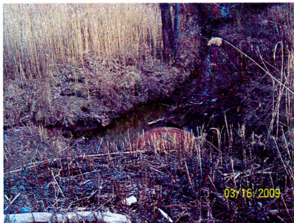
95 Culvert at Mautz Road looking east
