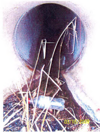
84 Culvert at Deer Road; about 18 inch culvert
