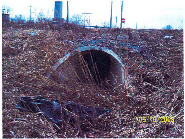
82 Culvert at Deer Road looking west
