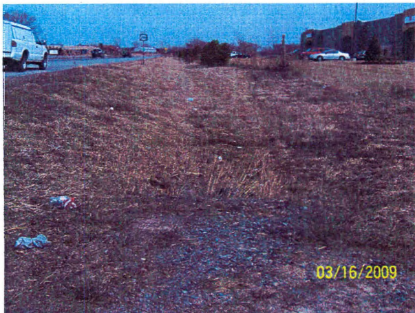
85 Drainage ditch leading to Deer Road culvert
