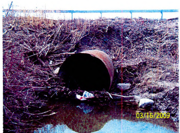
91 Culvert at Mautz Road looking west
