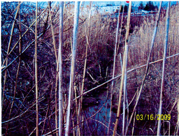
92 North drainage to culvert area
