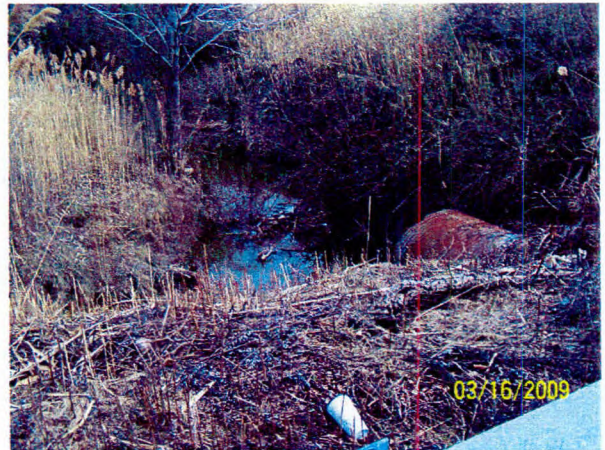
93 Culvert at Mautz Road looking east
