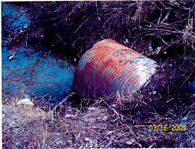
86 Culvert at Mautz Road looking east
