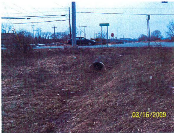
81 Culvert at Deer Road looking west
