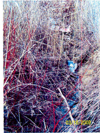
87 Drainage from culvert crossing Thompson Road from North; ~ 18 inch diameter
