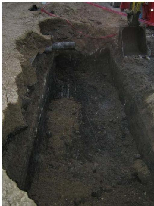
The vault was backfilled with clean soil from the Pond #2 excavation stockpile. Information on this soil can be found in the *Soils Management Report* submitted to NYSDEC on January 4, 2012.
