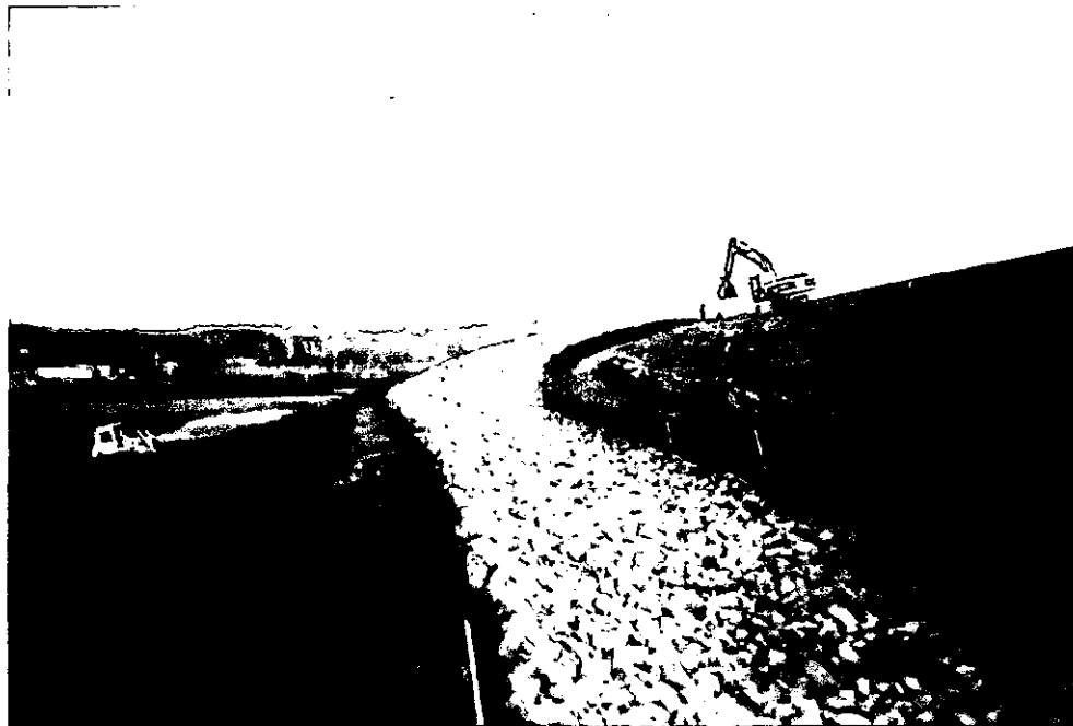
Photograph 26: Riprap placement in drainage swale and sand drainage layer of landfill. Photo looks east.
