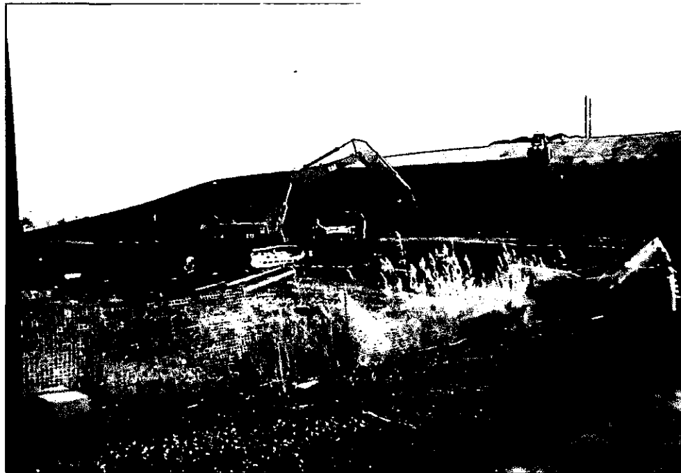
Photograph 24: Installation of barrier protection layer on landfill. Photo looks southeast.
