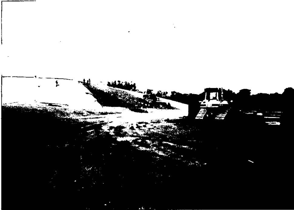
Photograph 21: Placement of geotextile and geomembrane on southern portion of landfill cap. Photo looks north.
