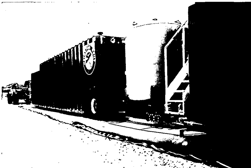
Photograph 5: Temporary wastewater treatment system consisting of Frac tanks and sand filter.
