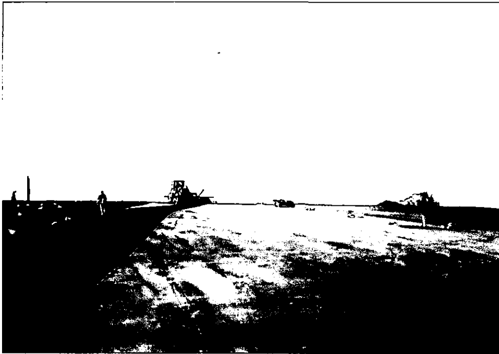
Photograph 20: Placement of geotextile on prepared landfill subgrade. Photo looks south.
