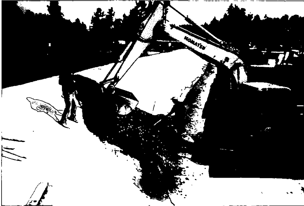
Photograph 29: Placement of gravel over GCL on new wastewater settling pond side slopes. Note weir in the background. Photo looks east.
