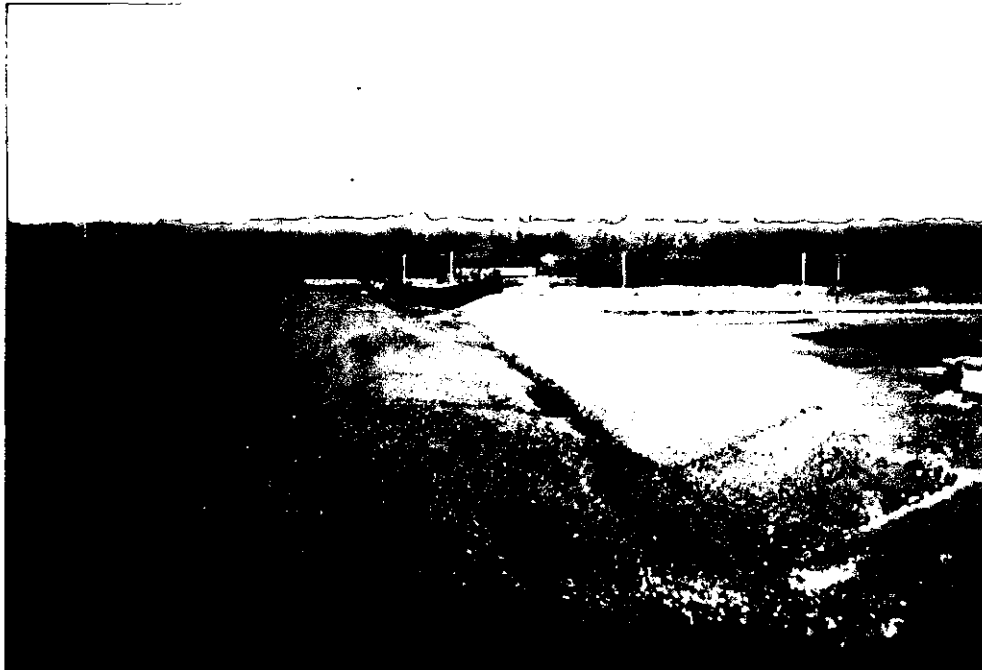
Photograph 25: Geotextile placement in drainage swale along eastern of landfill. Photo looks north.
