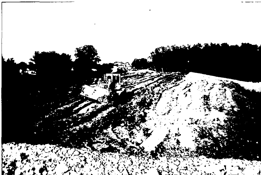
Photograph 16: Waste placement and consolidation on the landfill. Photo looks southeast.
