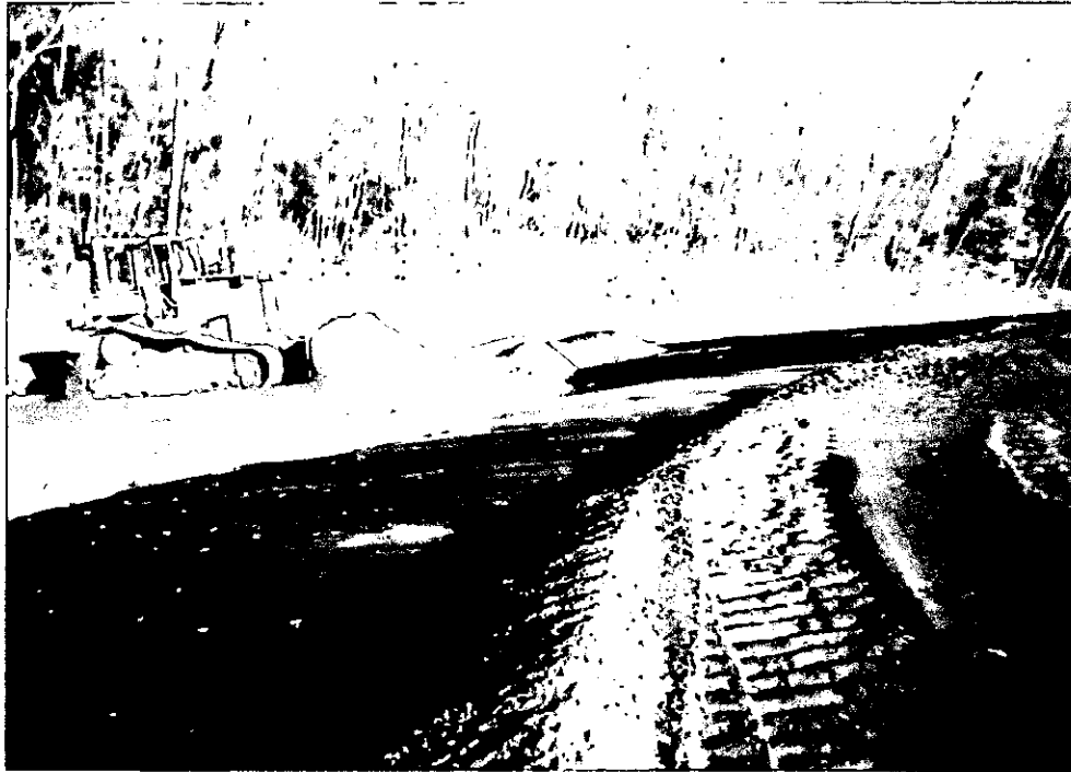
Photograph 23: Installation of sand drainage layer over geomembrane. Photo looks west.
