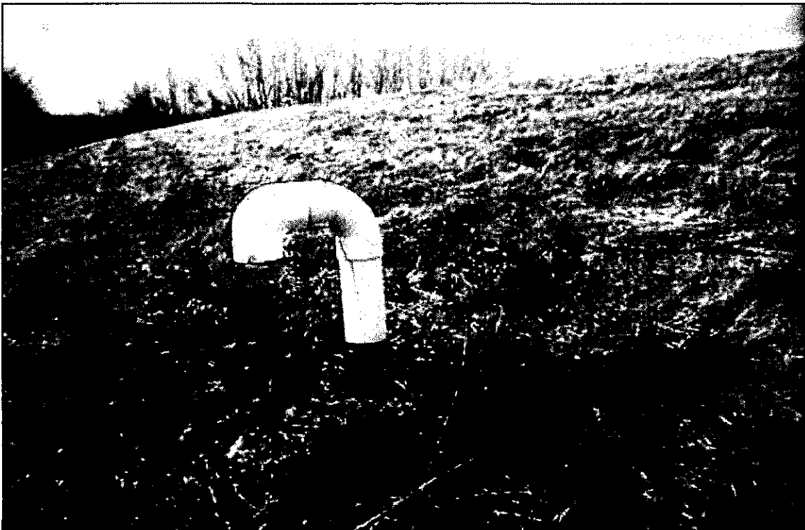
Photo 4: Typical landfill gas vent.
