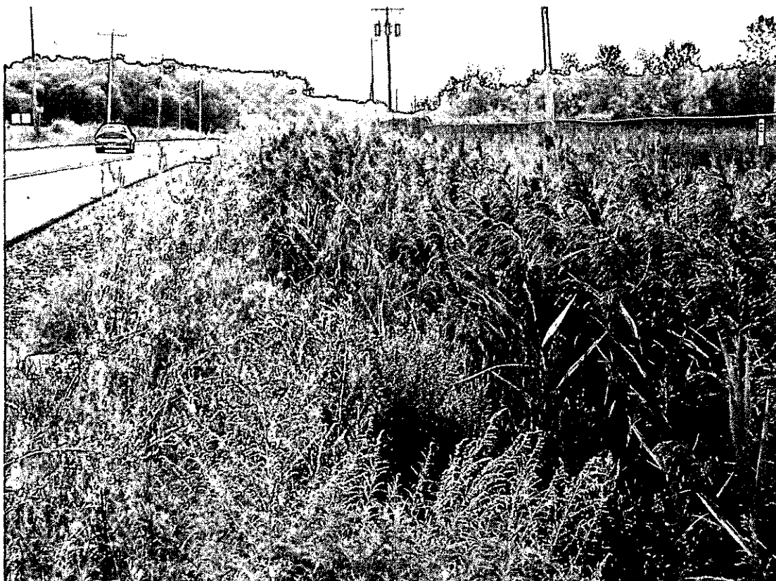
Photo 8: Northern portion of the fence along Factory Avenue. Photo looks east.
