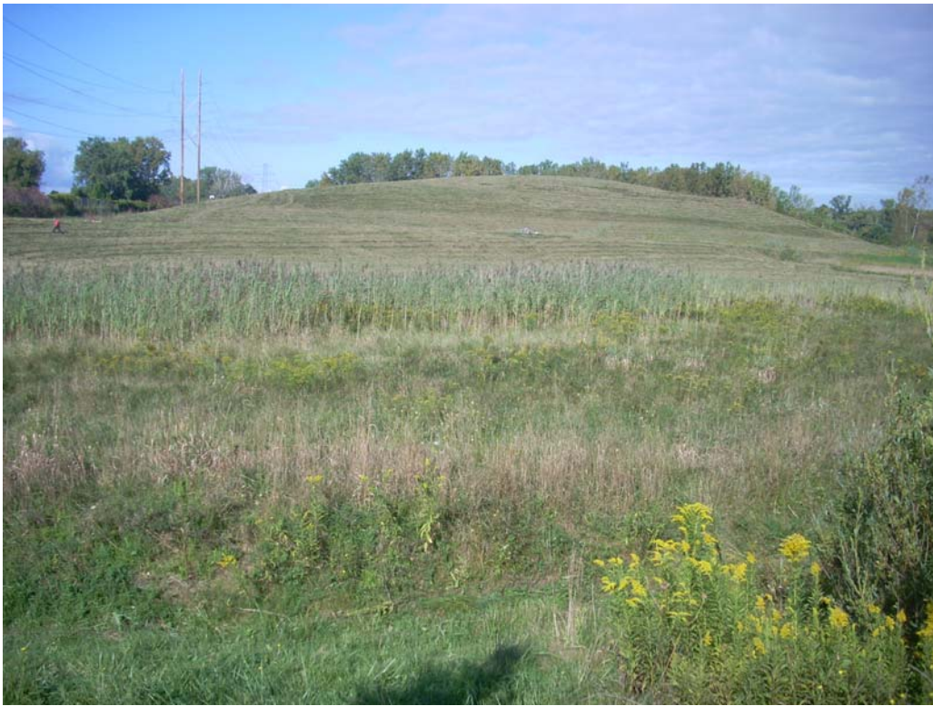
Photo 5: View of cut landfill facing west.
