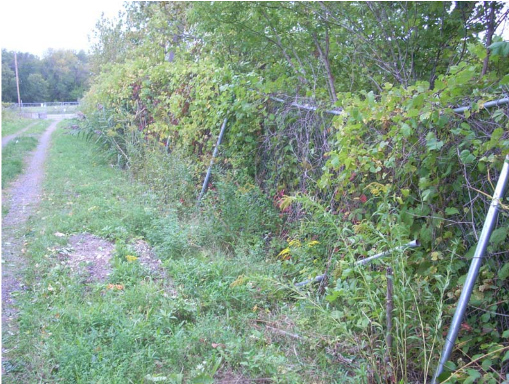
Photo 2: View of downed fencing along access road facing north.
