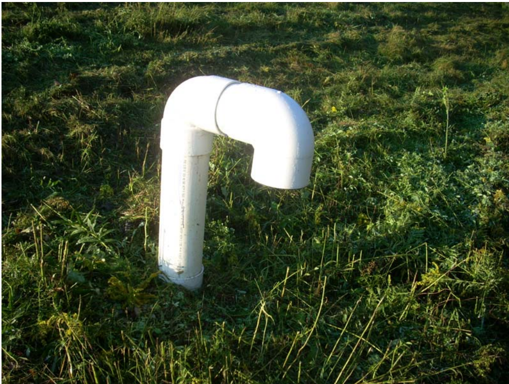
Photo 8: View of repaired landfill vent.
