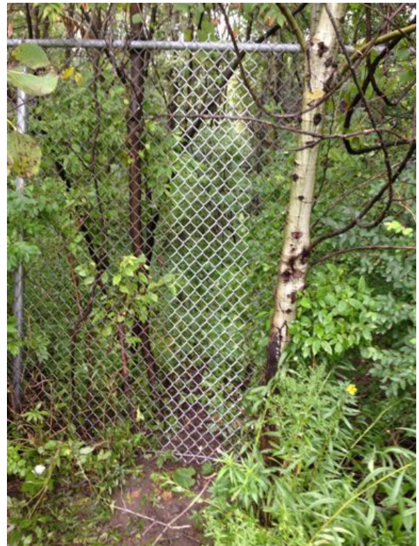
Fence Repair: West Fence Line
