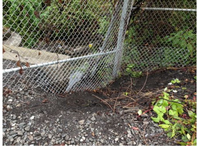
South Fence Line Vegetation Removal/fence improvement
