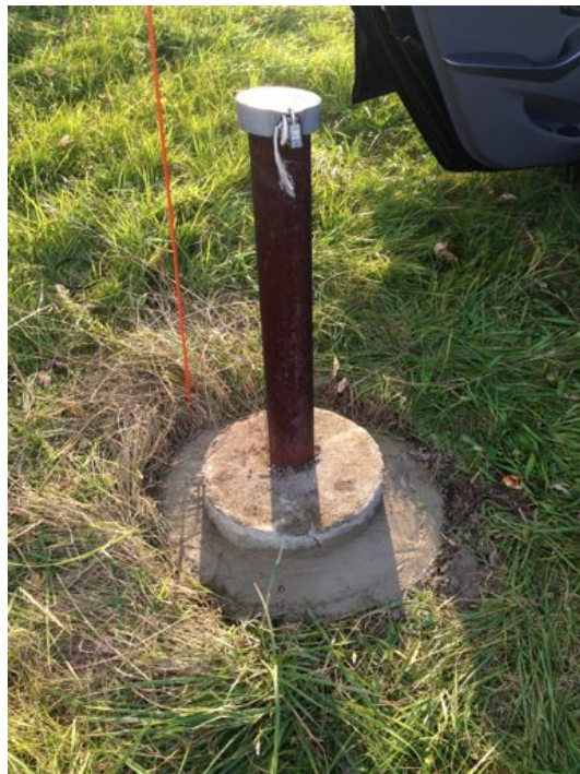
Monitoring Well MW-6: Pad Repair
