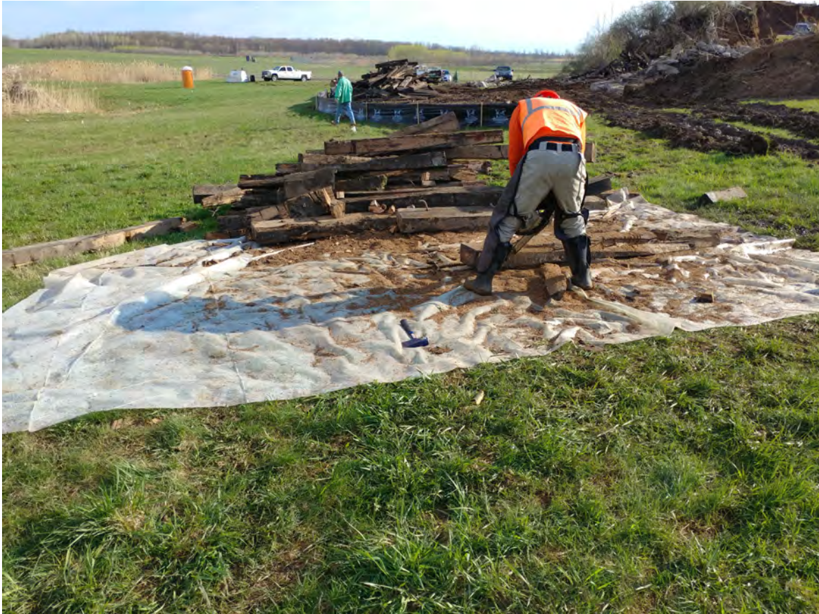
Using chainsaw to cut wood timbers to facilitate removal of MC/MD
