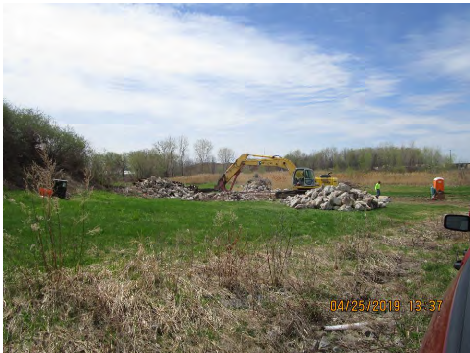
Staging of concrete in preparation for removal
