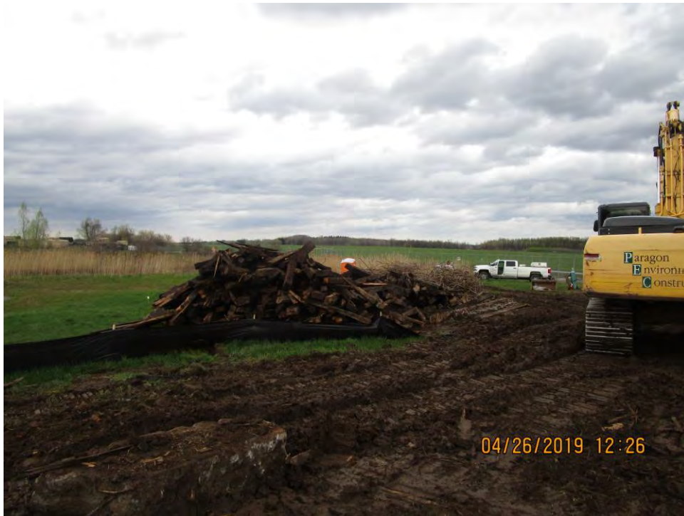
Timbers staged for removal to landfill
