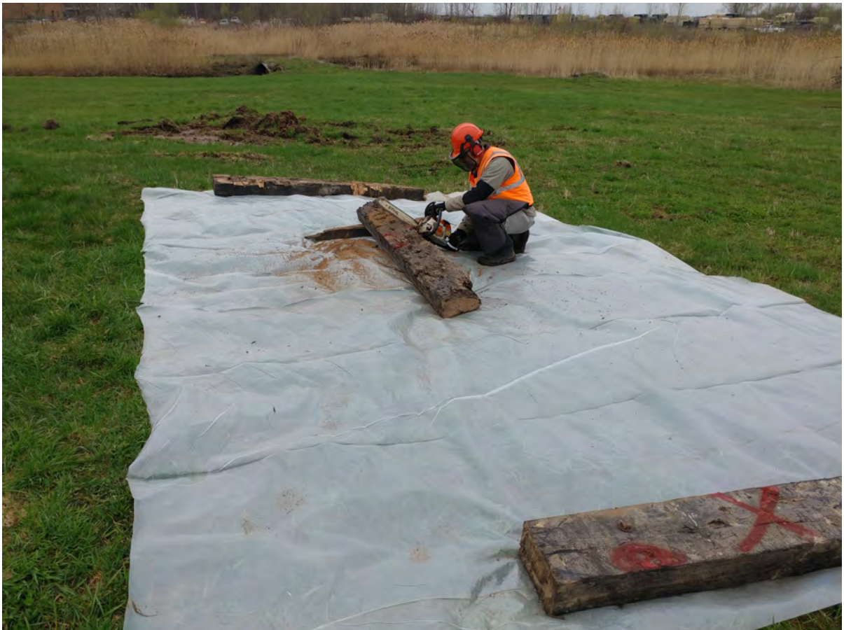
Preparing chainsaw for use in removing MC/MD
