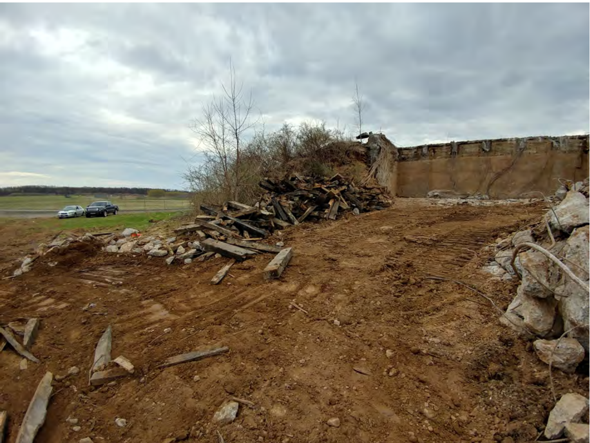
Remaining wood pile to be inspected
