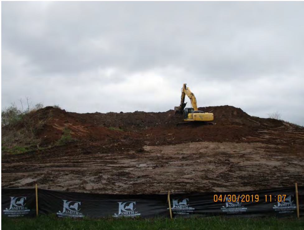
Collapsing the berm that surrounded the former firing-in buttress
