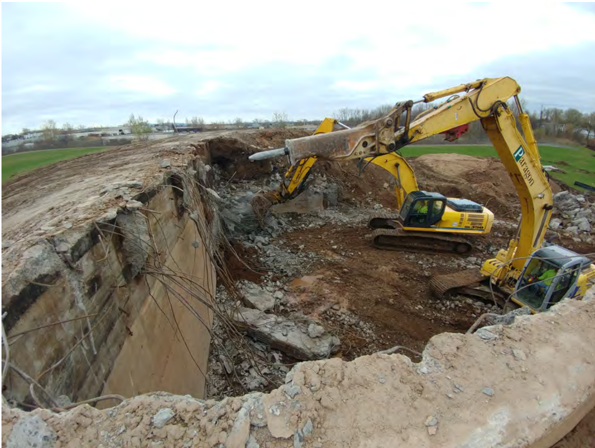
Jackhammer in use on concrete, removing via excavator
