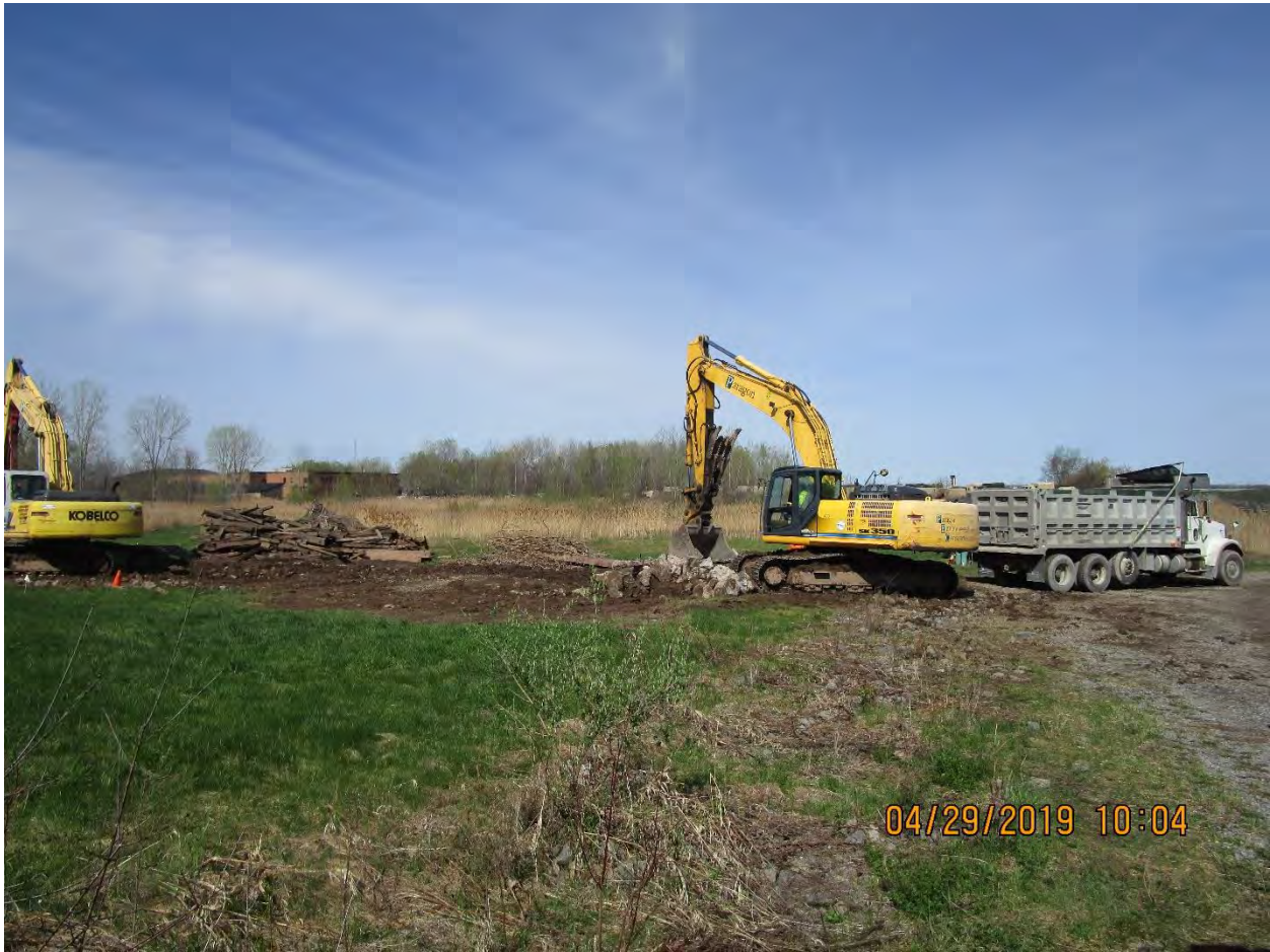
Loading a dump truck with concrete for removal off-site
