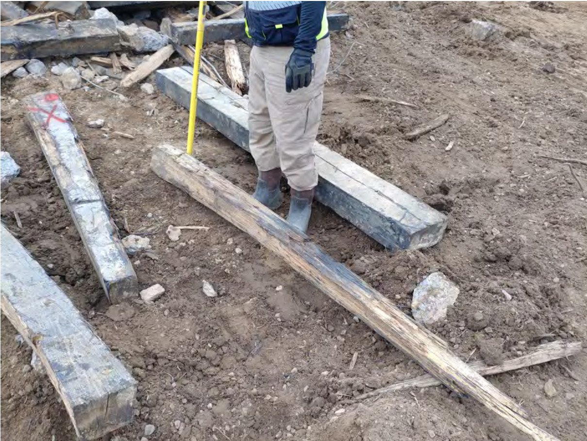
Inspecting wood timbers via magnetic locator
