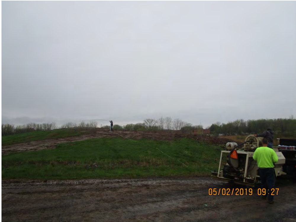
Tim Murphy Landscaping beginning to hydroseed from the top of the hill
