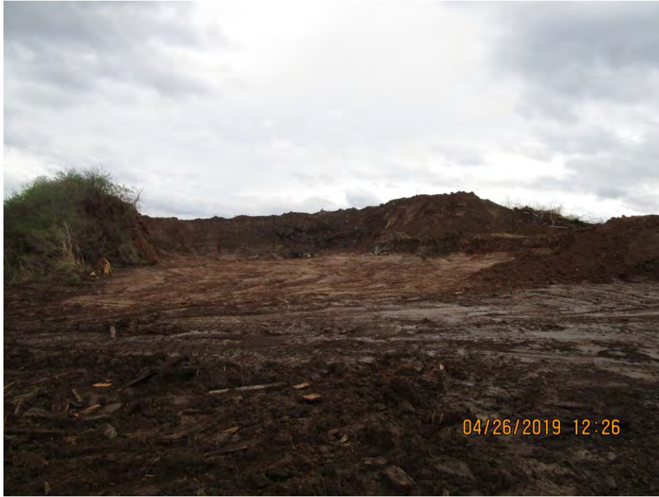
All demolition debris clear of demolition area
