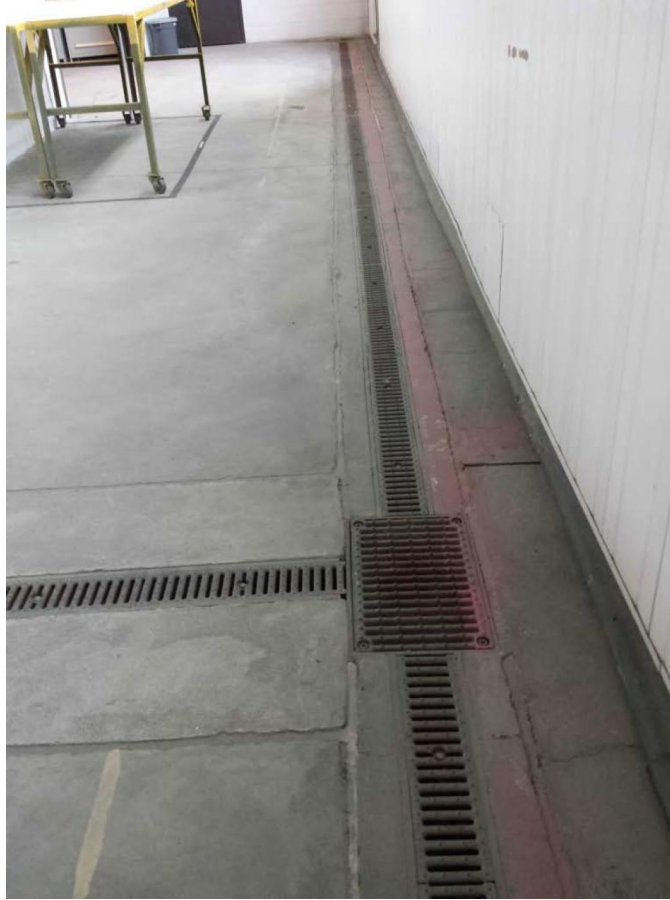
Photo 6: Trench drains were observed in Building 646, which historically had an AFFF fire suppression system.
