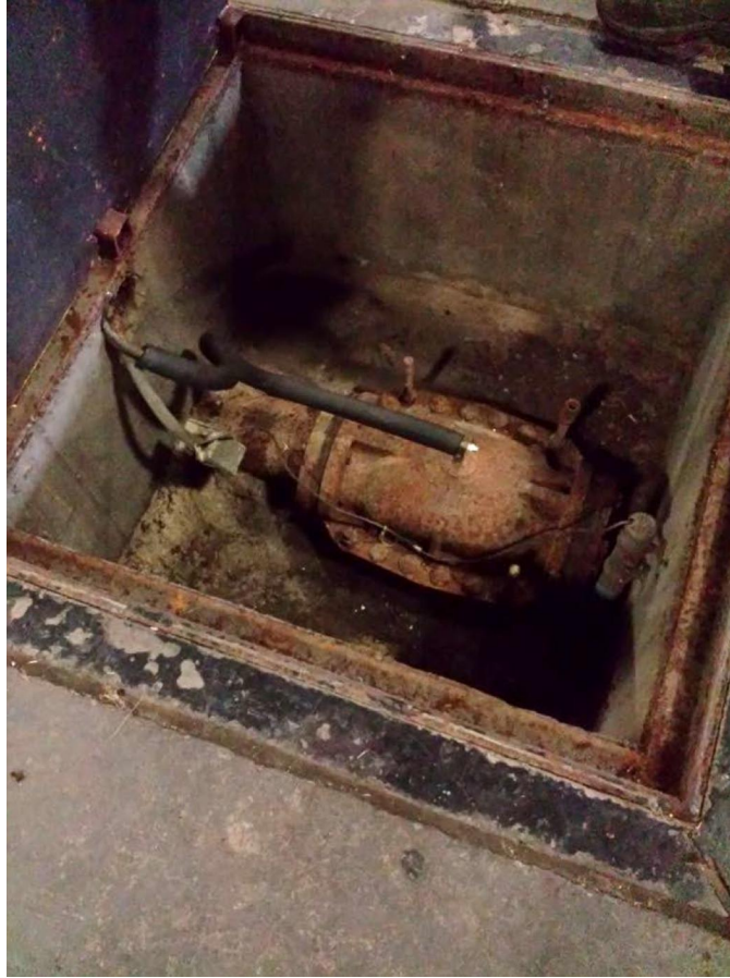
Photo 7: A drain/valve system was located in the center of Building 618. No other floor drains were present. Building 618 was historically equipped with an AFFF fire suppressions system.
